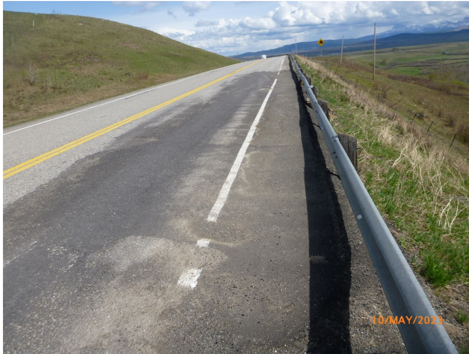
Photo 4 Cracking on the west shoulder of the highway outside of patched area. Photo taken facing southeast on May 10, 2023.
