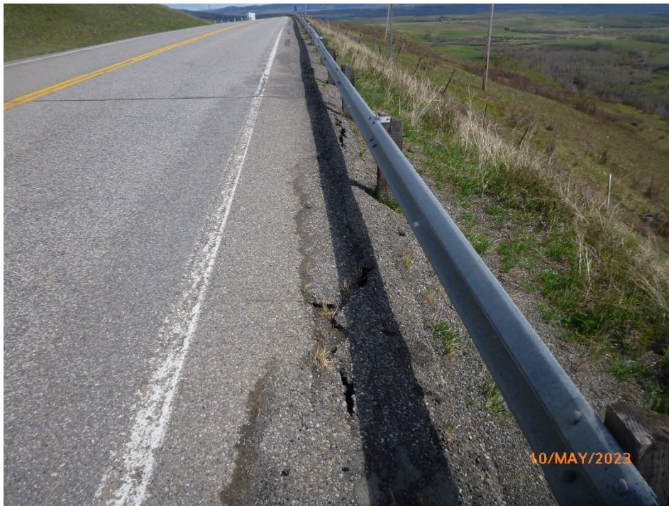
Photo 4 Cracking on the west shoulder of the highway outside of patched area. Photo taken facing southeast on May 10, 2023.
