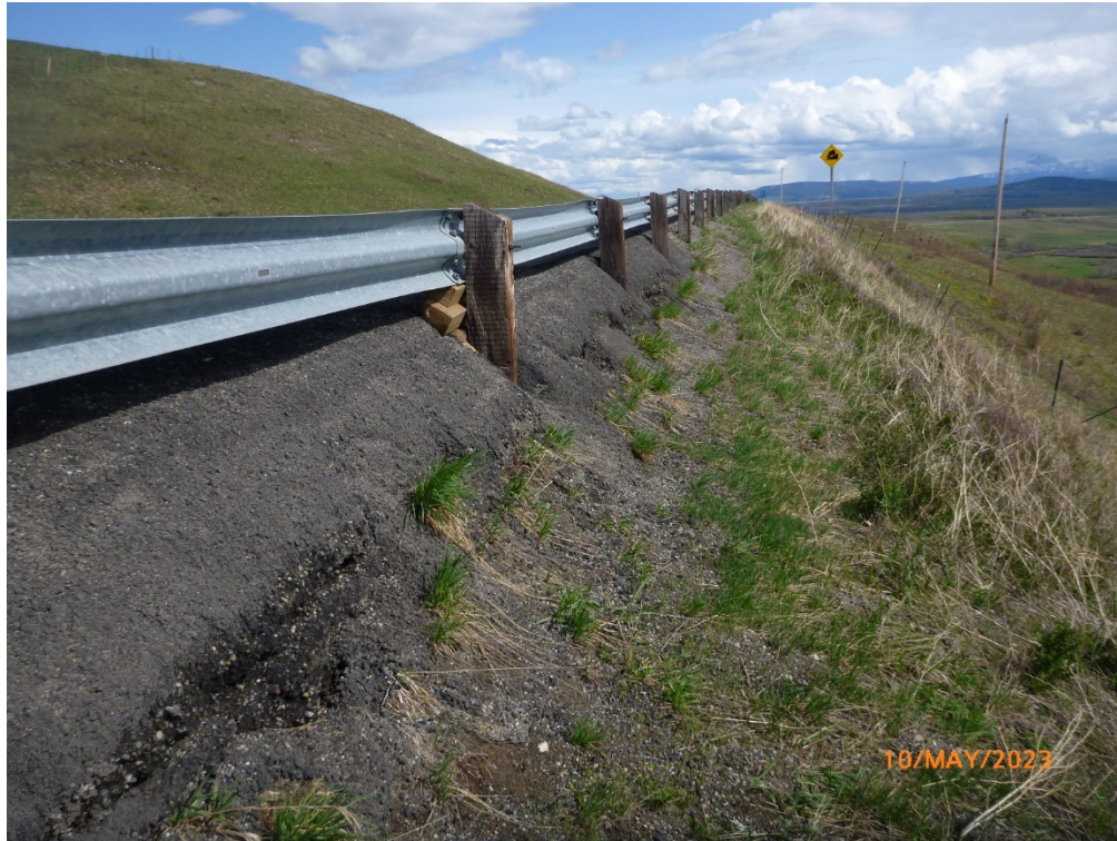
Photo 5 Up to 1.2 m of asphalt on west shoulder. Photo taken facing southeast on May 10, 2023.
