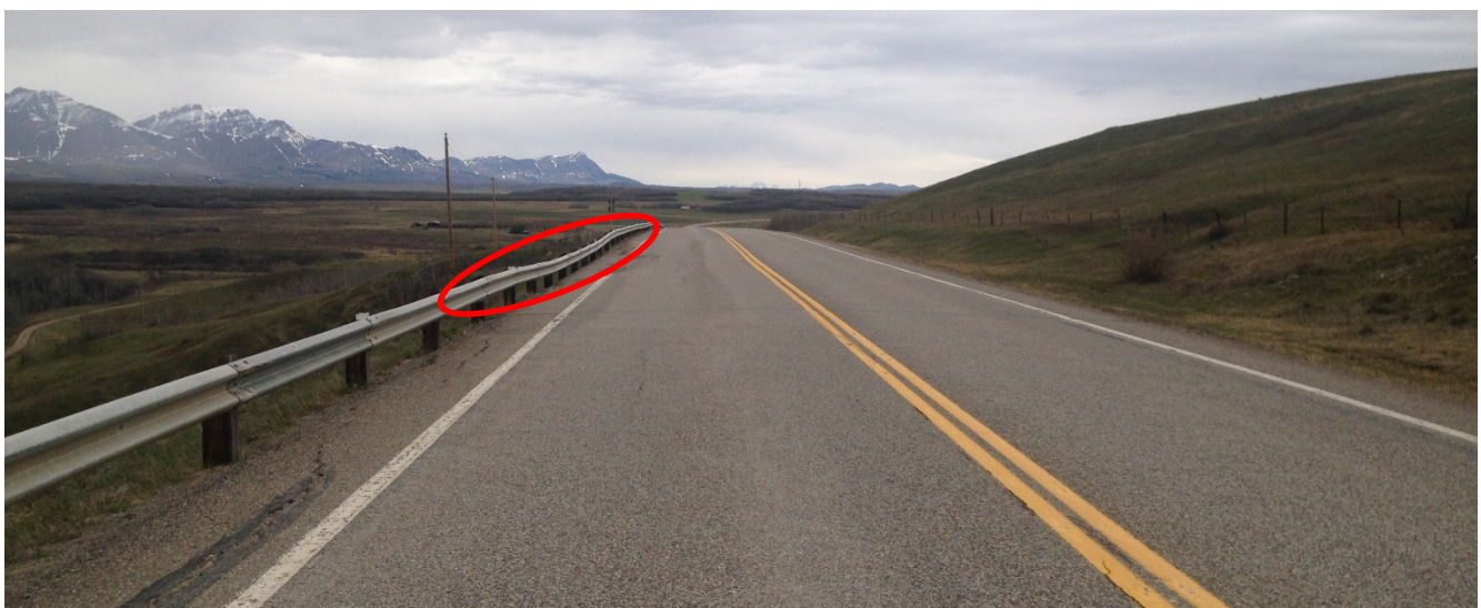
Photo 2 Dip in guard rail (red circle) due to slope movement. Photo was taken facing northwest on May 10, 2019.
