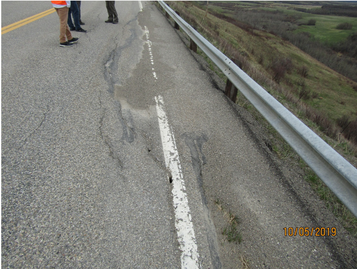
Photo 2 Dip in guard rail (red circle) due to slope movement. Photo was taken facing northwest on May 10, 2019.
