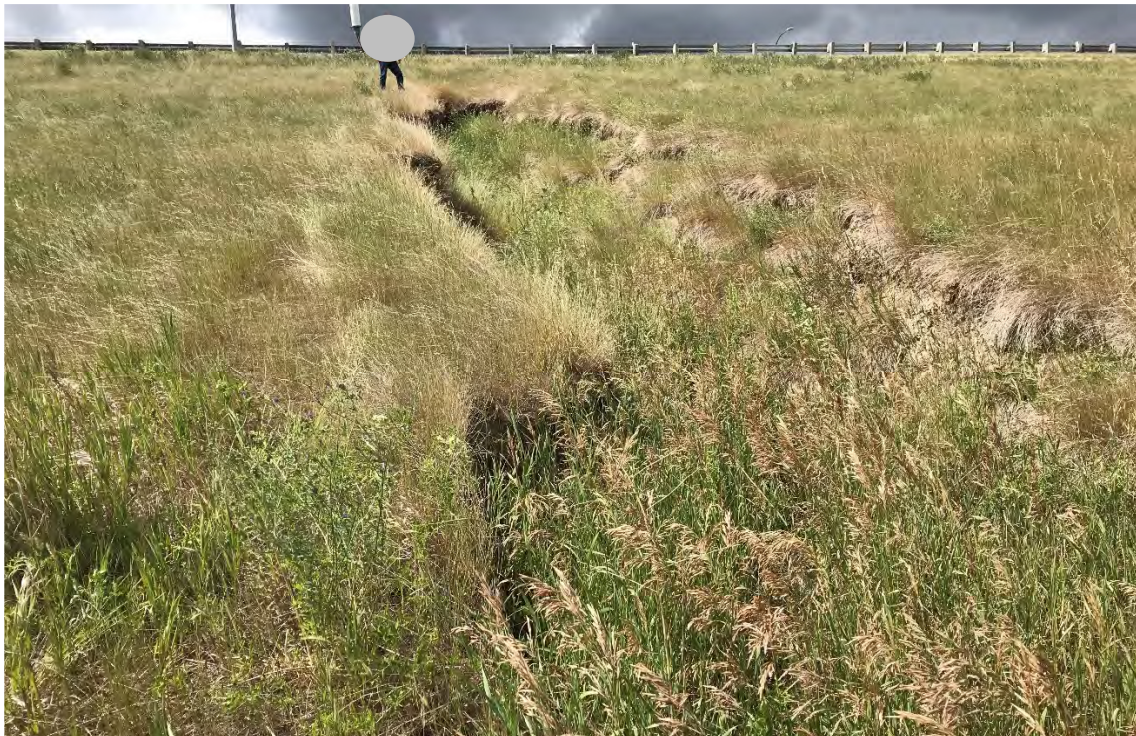
Photo 2 Surface runoff erosion gully viewed from lower part of the embankment. Photo was taken facing west on July 8, 2021.
