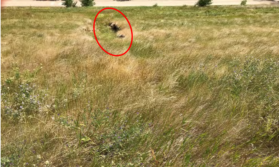
Photo 2 Surface runoff erosion gully viewed from lower part of the embankment. Photo was taken facing west on July 8, 2021.
