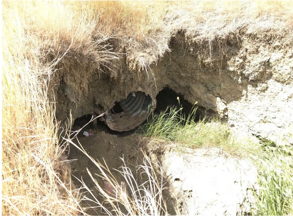
Photo 4 Possible sinkhole forming near crest of slope, near to a utility box. Photo taken facing south on July 8, 2021.
