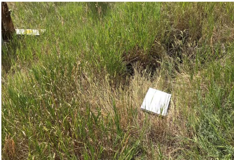
Photo 4 Possible sinkhole forming near crest of slope, near to a utility box. Photo taken facing south on July 8, 2021.
