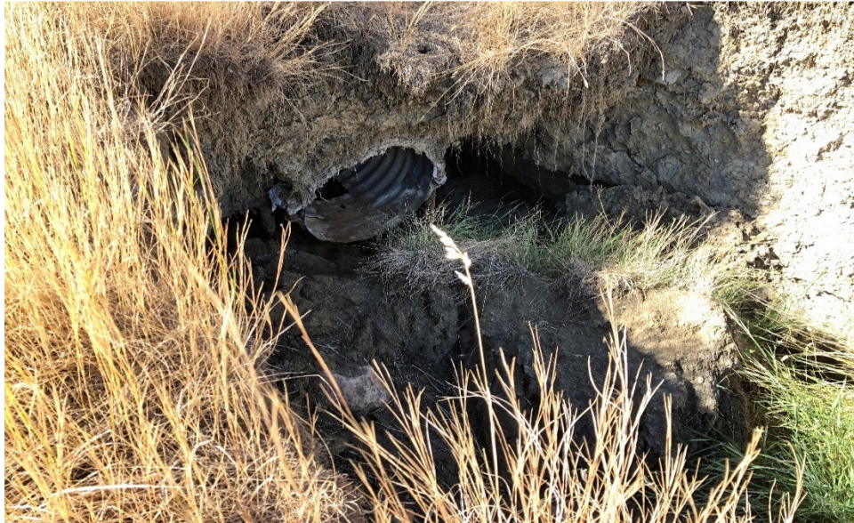
Photo 8 The CSP culvert has rusted over time and separated at joints, causing the erosion gully to retrogress up the slope. Photo taken facing southwest on September 9, 2020.
