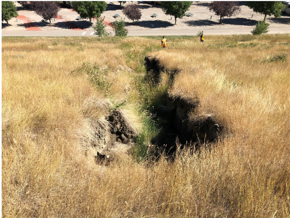
Photo 10 Surface runoff erosion gully viewed from midway down the embankment. Photo was taken facing west on September 9, 2020.
