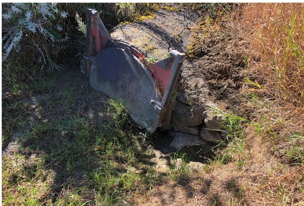
Photo 12 The flap valve is bolted open, but the outflow channel has silted up due to sediment from the west side of the highway washing through the underdrain culvert.
