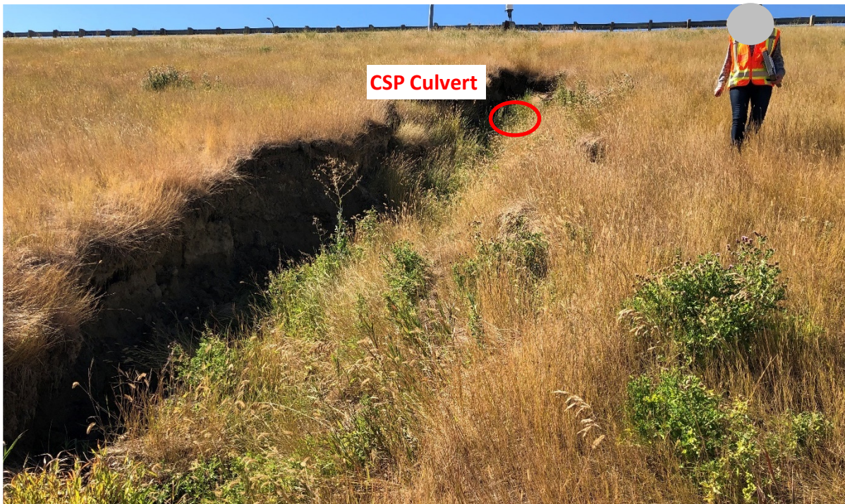
Photo 10 Surface runoff erosion gully viewed from midway down the embankment. Photo was taken facing west on September 9, 2020.
