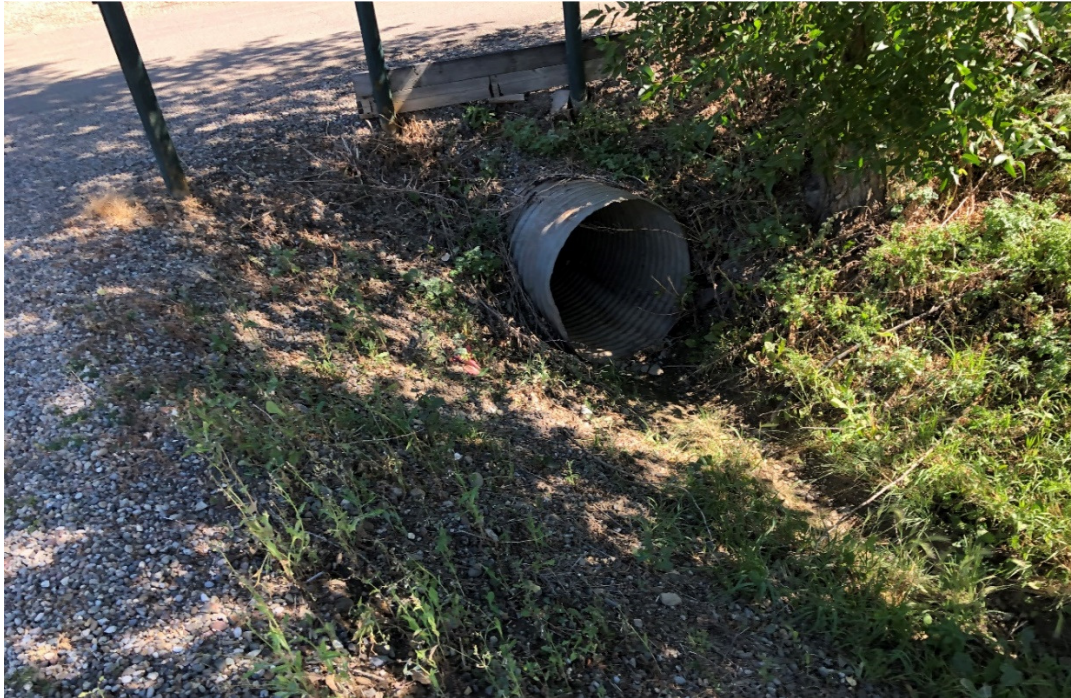
Photo 18 Overgrown drainage channel between the CSP culvert and the river. Photo taken on September 9, 2020.
