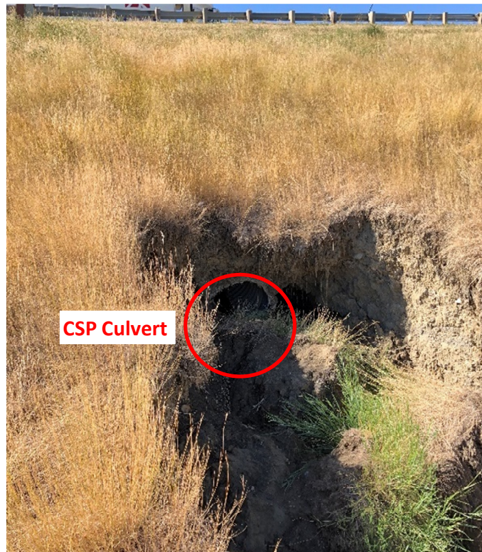
Photo 8 The CSP culvert has rusted over time and separated at joints, causing the erosion gully to retrogress up the slope. Photo taken facing southwest on September 9, 2020.
