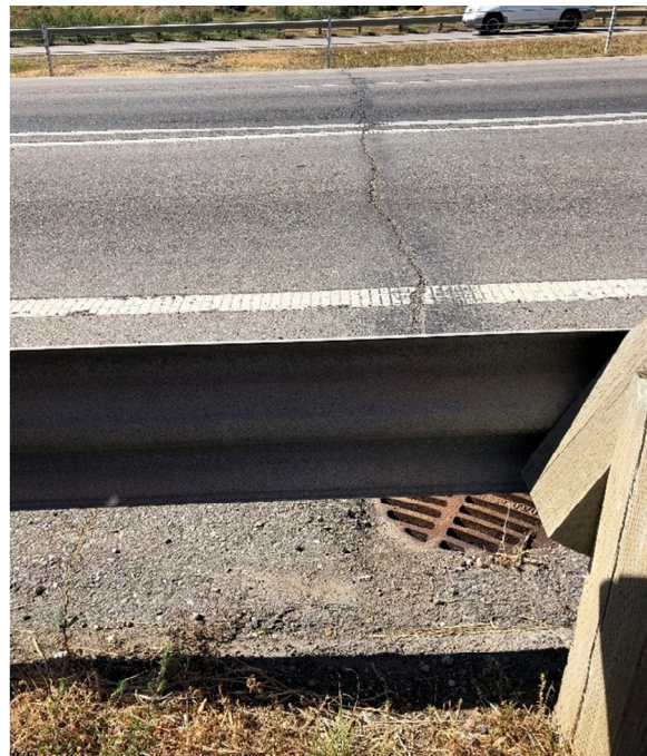
Photo 2 Crack in pavement surface over highway drainage. Photo taken facing southwest on September 9, 2020.
