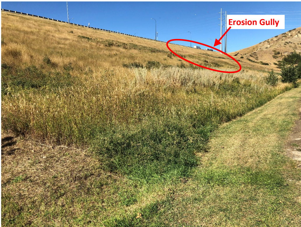
Photo 6 Highway embankment from toe of slope. Photo taken facing southeast from the RV Park on September 9, 2020.
