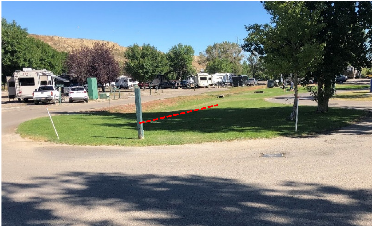
Photo 14 Shallow open drainage channel from the underdrain pipe to the river (red dashed line). Photo taken facing north on September 9, 2020.
