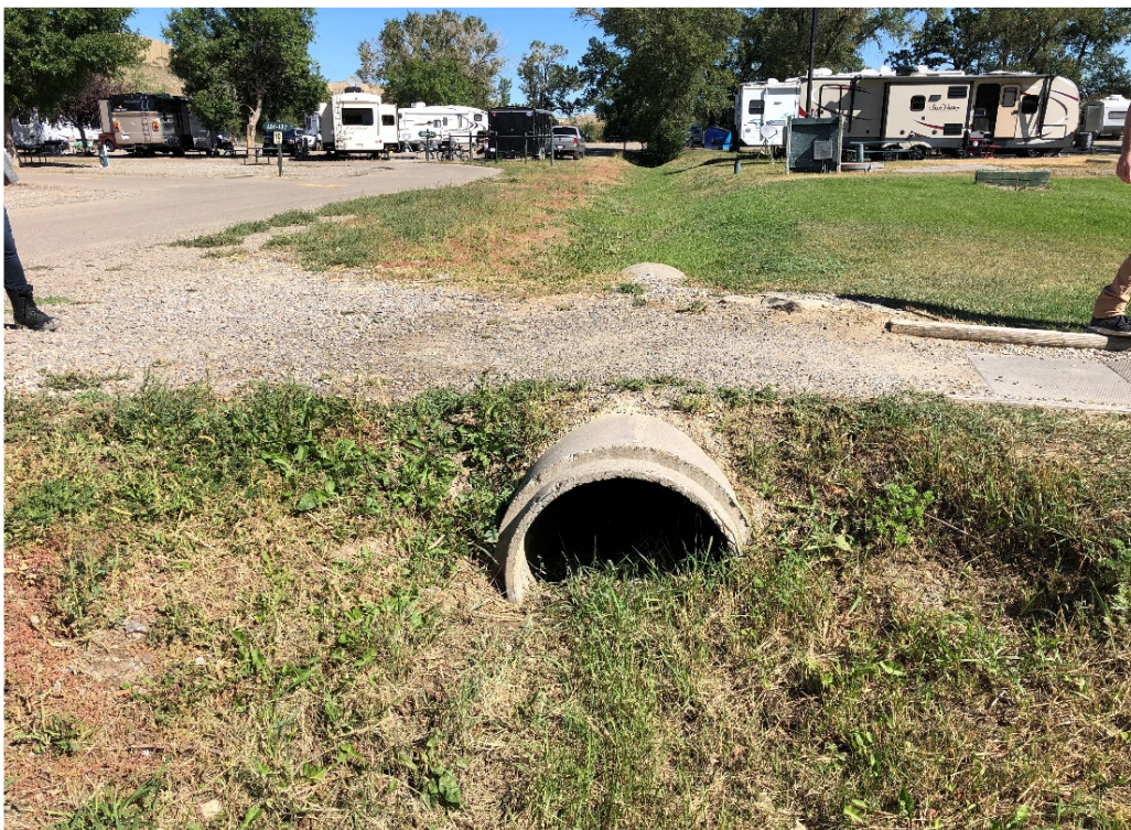
Photo 16 Shallow drainage channel from the concrete underdrain to the river. Several silted up culverts are located along the drainage channel which contributes to overland flooding in the RV Park. Photo taken facing northeast on September 9, 2020.
