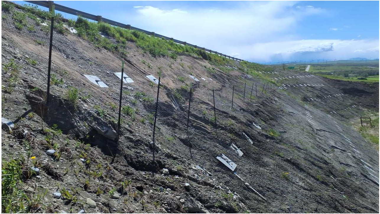
Photo 4 Slope movement. Material moving around soil nail anchor plates. Photo taken facing south on May 29, 2024.
