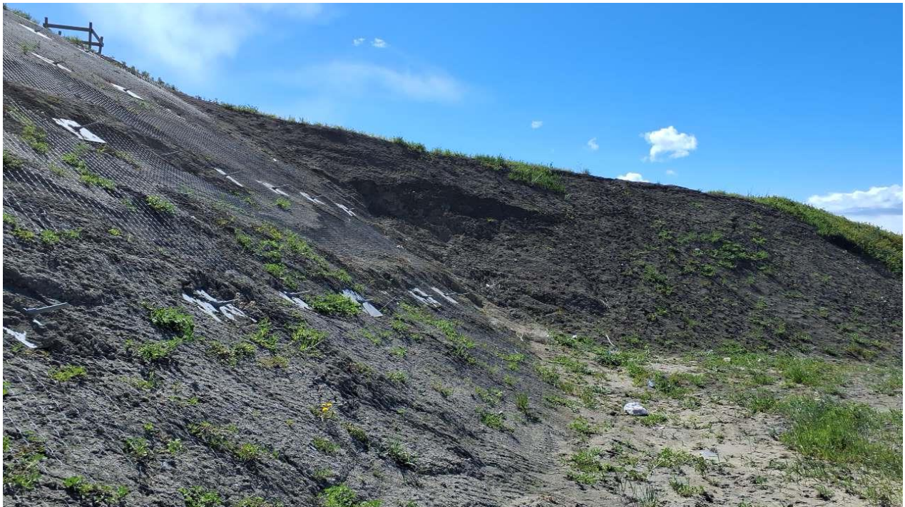
Photo 6 Slope movement on west flank of repair slope. Photo taken facing northeast on May 29, 2024.
