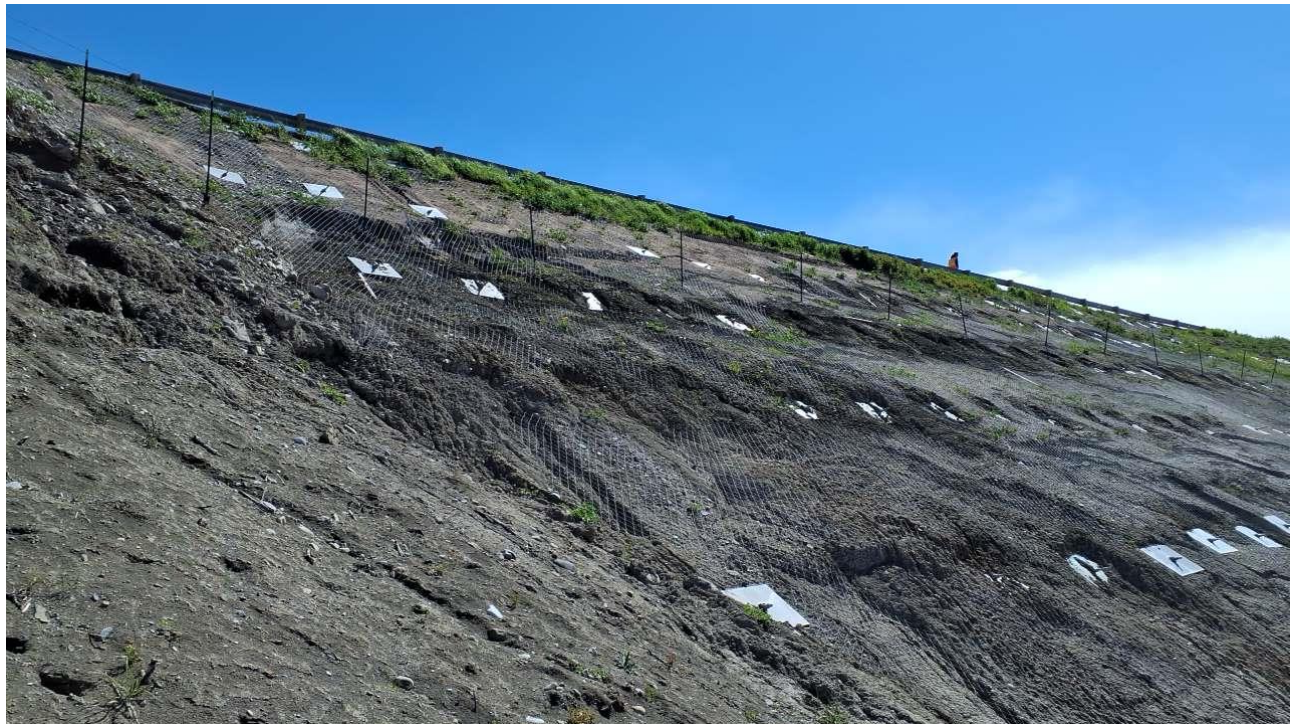
Photo 4 Slope movement. Material moving around soil nail anchor plates. Photo taken facing south on May 29, 2024.
