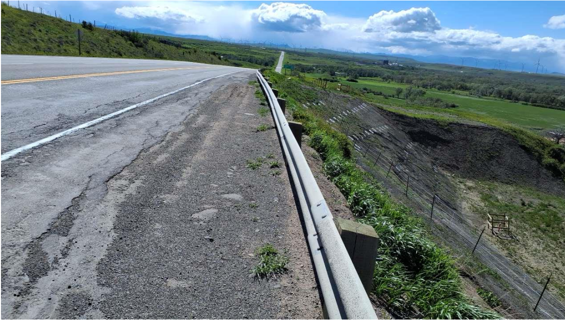
Photo 2 Erosion rilling from highway runoff down the slope. Photo taken on May 29, 2024 looking south.
