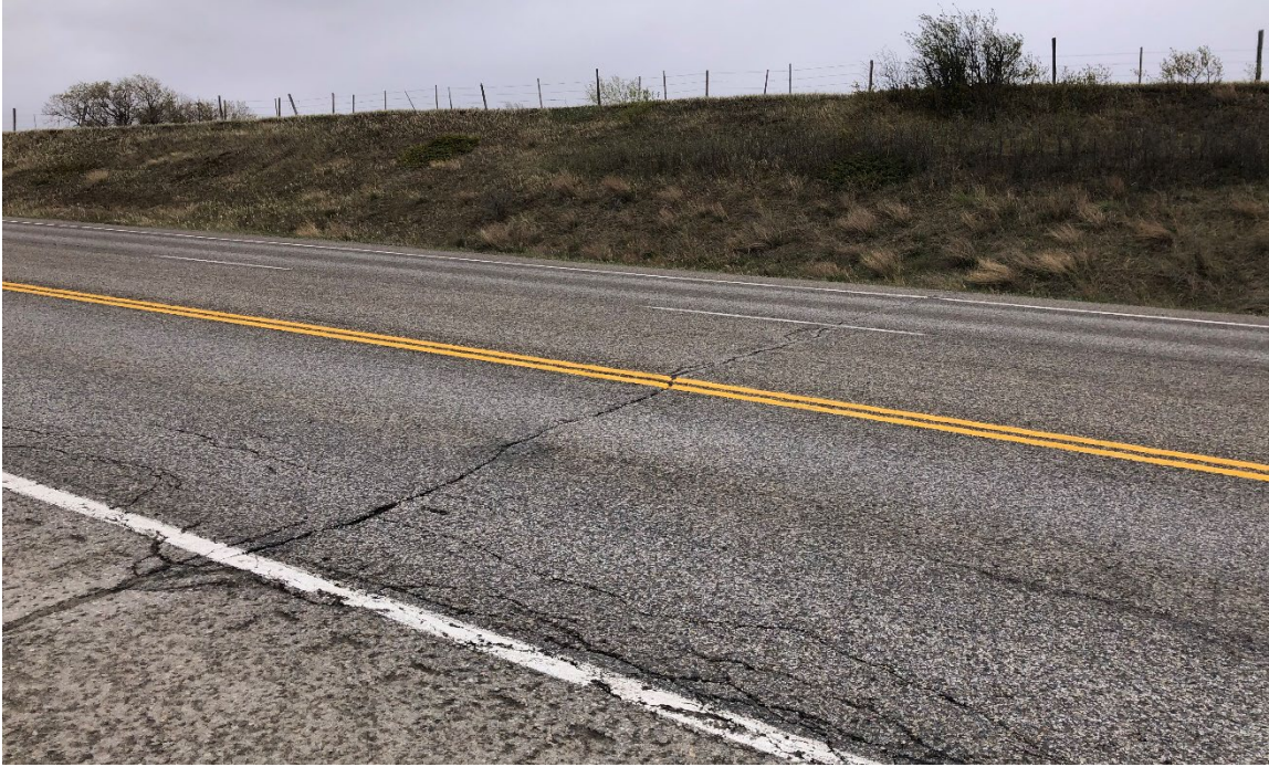
Photo 2 Slide movement is impacting the highway surface and has deformed (cracked and settled) the 2017 pavement patch. Photo taken May 19, 2022 facing east.
