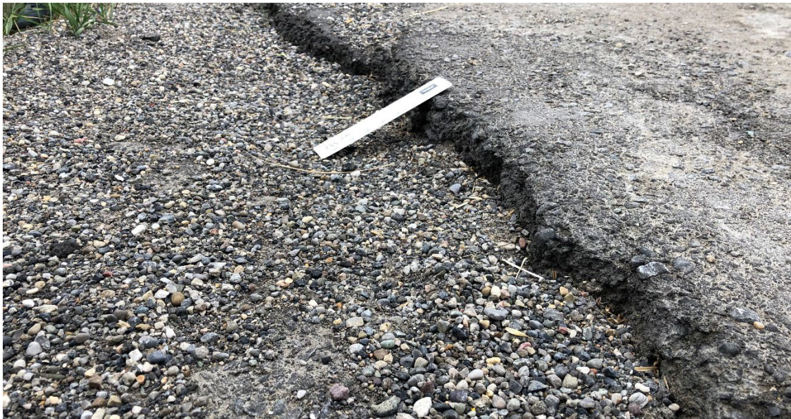
Photo 4 Pavement cracking and settlement in the 2017 pavement patch. Photo taken May 19, 2022, facing west.
