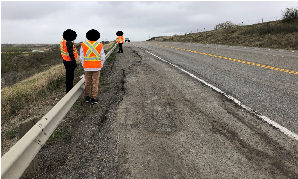
Photo 2 Slide movement is impacting the highway surface and has deformed (cracked and settled) the 2017 pavement patch. Photo taken May 19, 2022 facing east.
