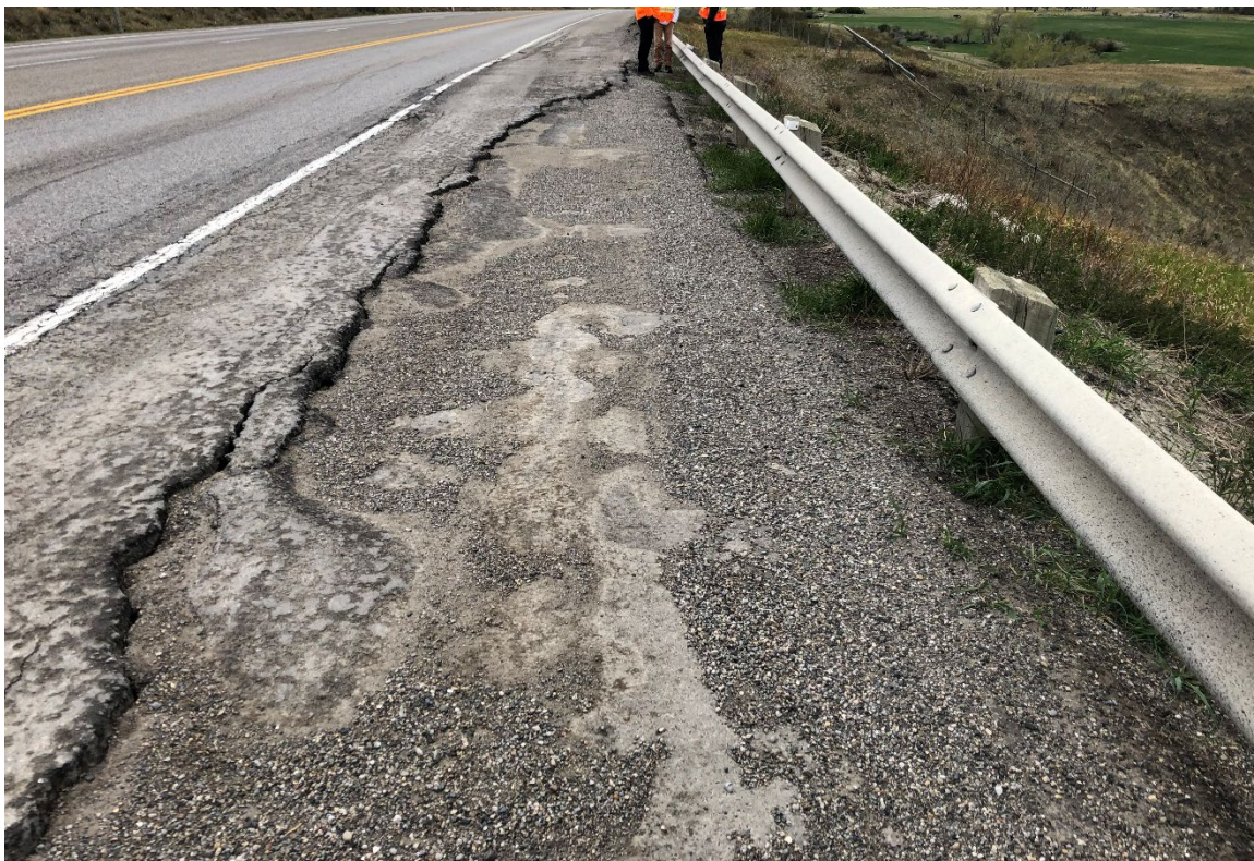
Photo 4 Pavement cracking and settlement in the 2017 pavement patch. Photo taken May 19, 2022, facing west.
