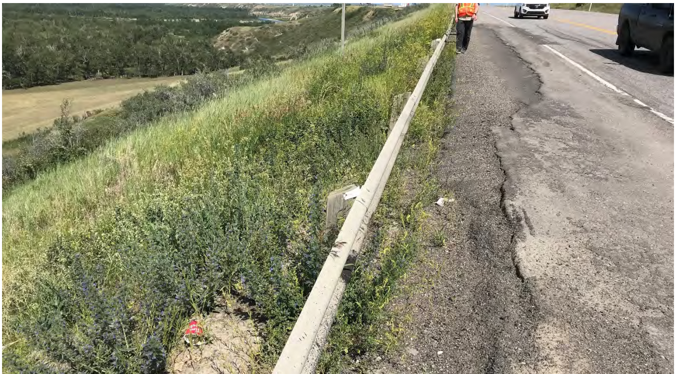
Photo 2 Site I - Head scarp impacting the highway. The 2017 patching has cracked and settled. Photo was taken facing east on July 8, 2021.
