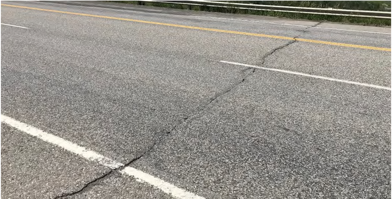
Photo 2 Site I - Head scarp impacting the highway. The 2017 patching has cracked and settled. Photo was taken facing east on July 8, 2021.
