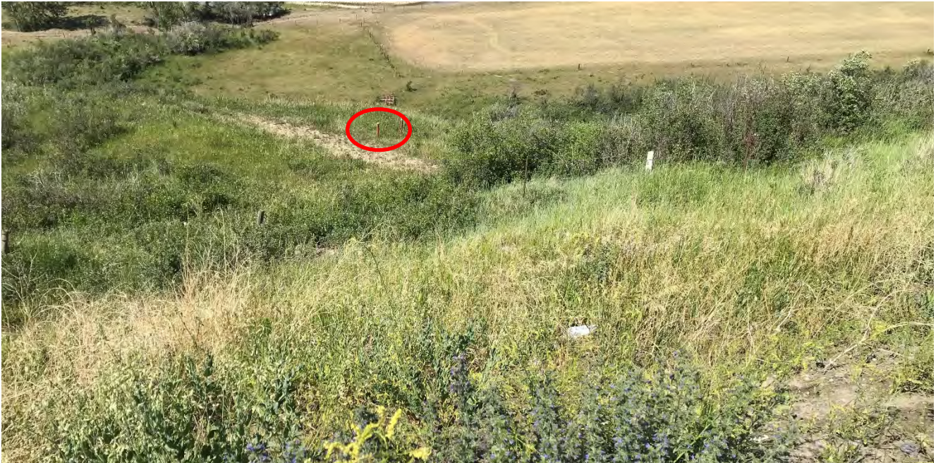
Photo 3 Site I - Instrumentation installed on a bench constructed mid slope in the middle of the slide area (red circle). Photo was taken facing northwest on July 8, 2021.
