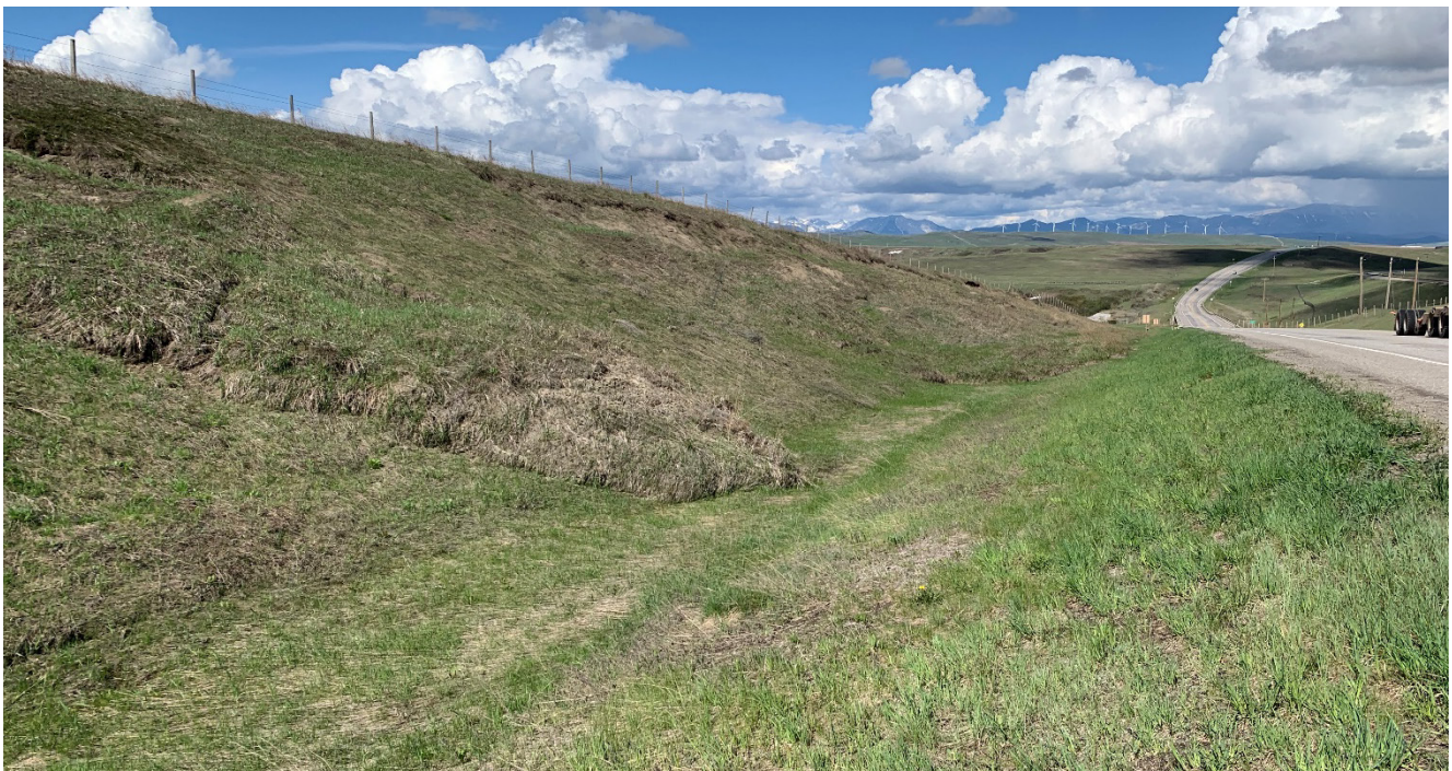
Photo 2 Toe rolls coalescing and blocking the ditch. Photo was taken facing west on May 10, 2023.
