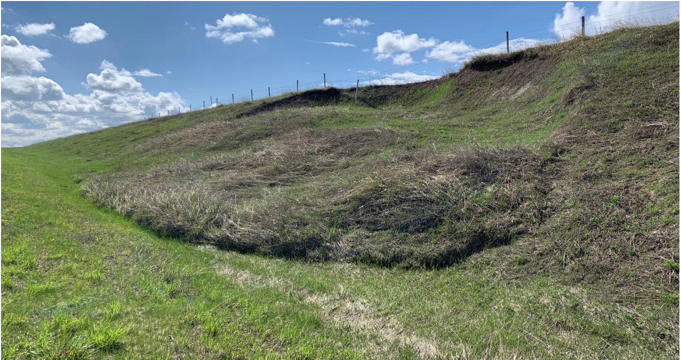
Photo 2 Toe rolls coalescing and blocking the ditch. Photo was taken facing west on May 10, 2023.
