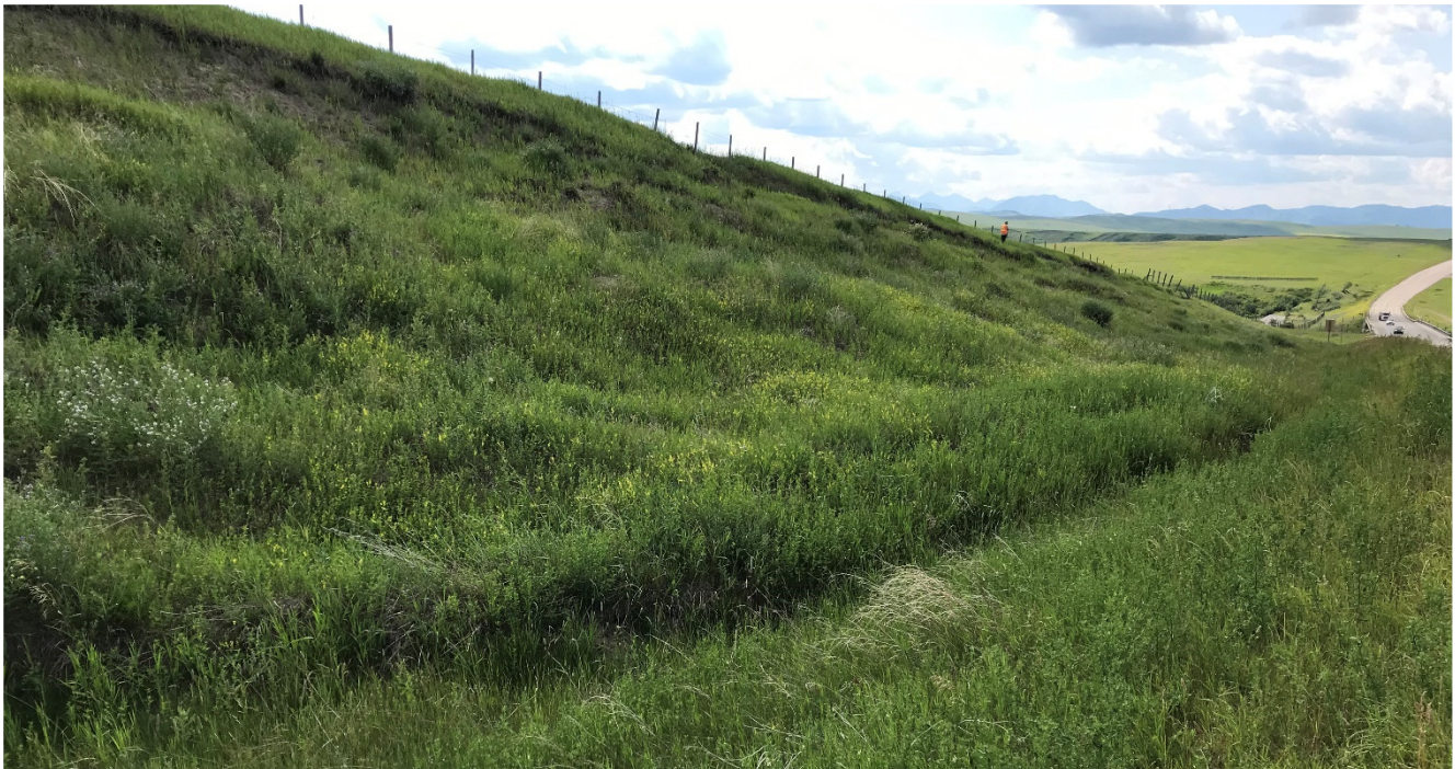
Photo 2 Toe rolls coalescing and blocking the ditch. Photo was taken facing west on July 8, 2021.
