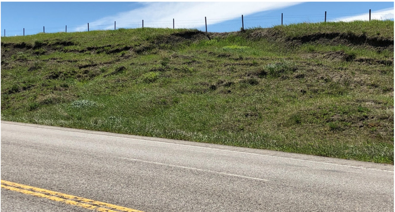
Photo 2 Looking south at the north-facing failing back slope. The photo was taken on June 9, 2020.
