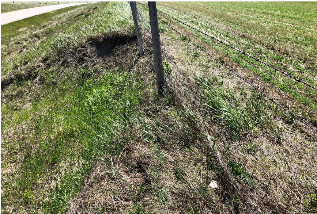
Photo 4 Fence being undermined in several locations by slope failure. Photo taken facing east on June 9, 2020.
