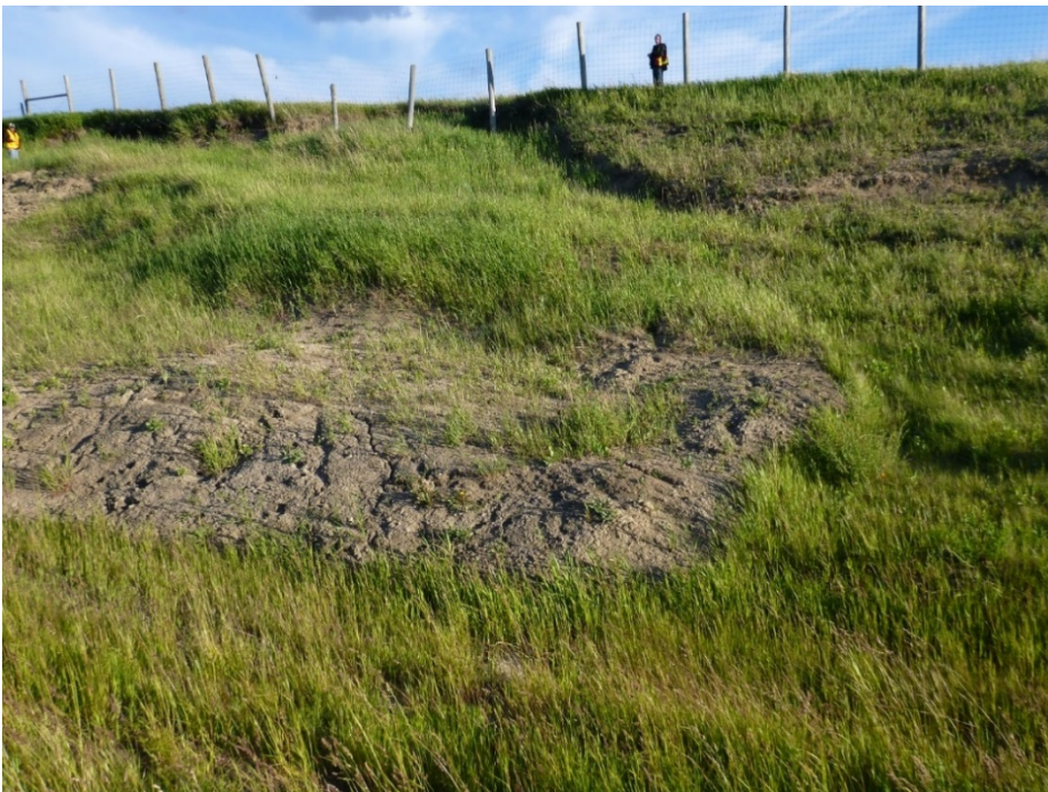
Photo 6 A closer look at the failing back slope. The fence has failed as a result of the failing slope. The photo was taken on June 15, 2016.
