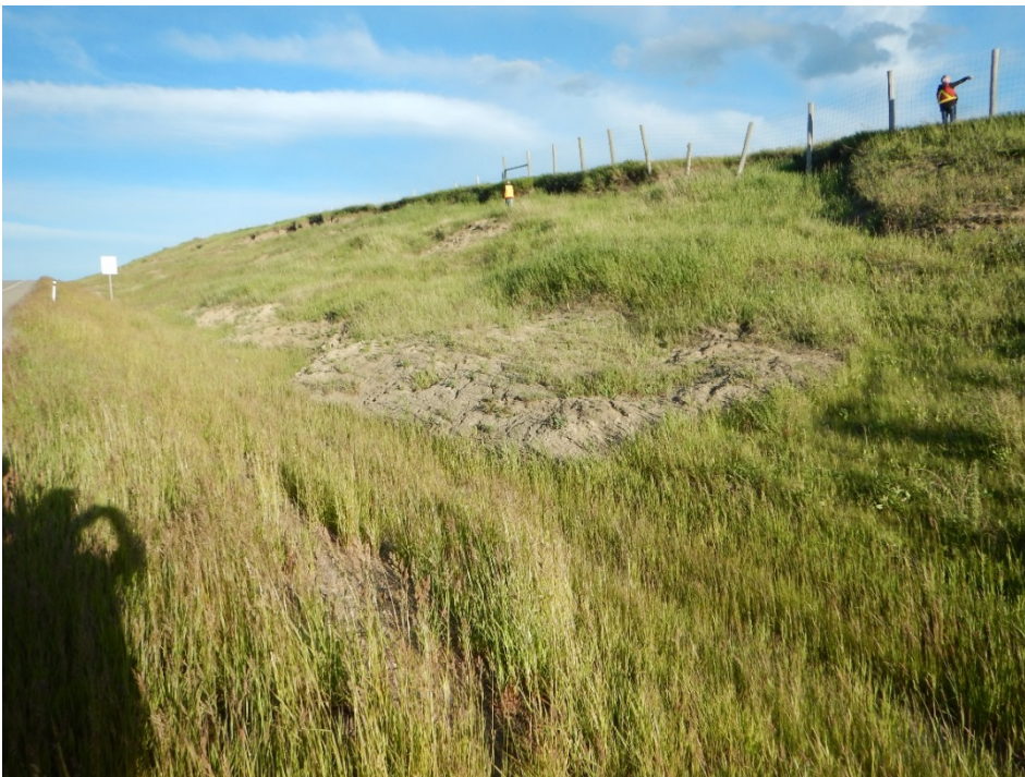
Photo 4 Looking southeast at the failing back slope. The photo was taken on June 15, 2016.
