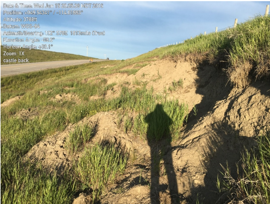
Photo 8 Looking east at the failing back slope approximately 200 m on the south side. Rills on the slope were present. Photo taken on June 15, 2016.
