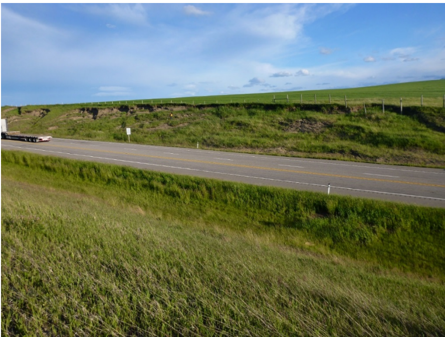
Photo 2 Looking south at the north-facing failing back slope. The photo was taken on June 15, 2016.
