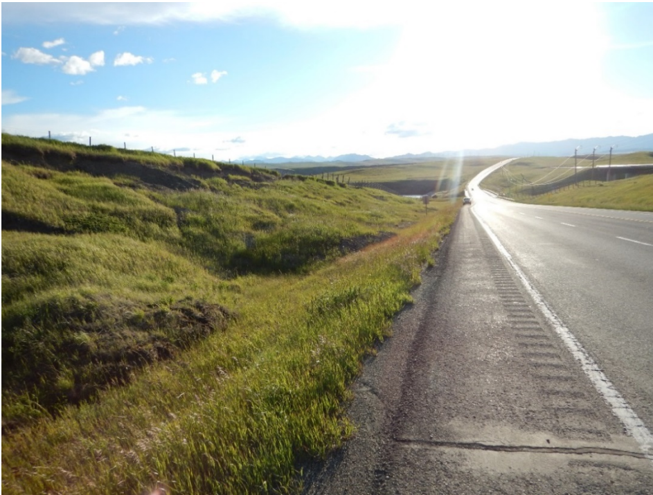
Photo 6 A closer look at the failing back slope. The fence has failed as a result of the failing slope. The photo was taken on June 15, 2016.
