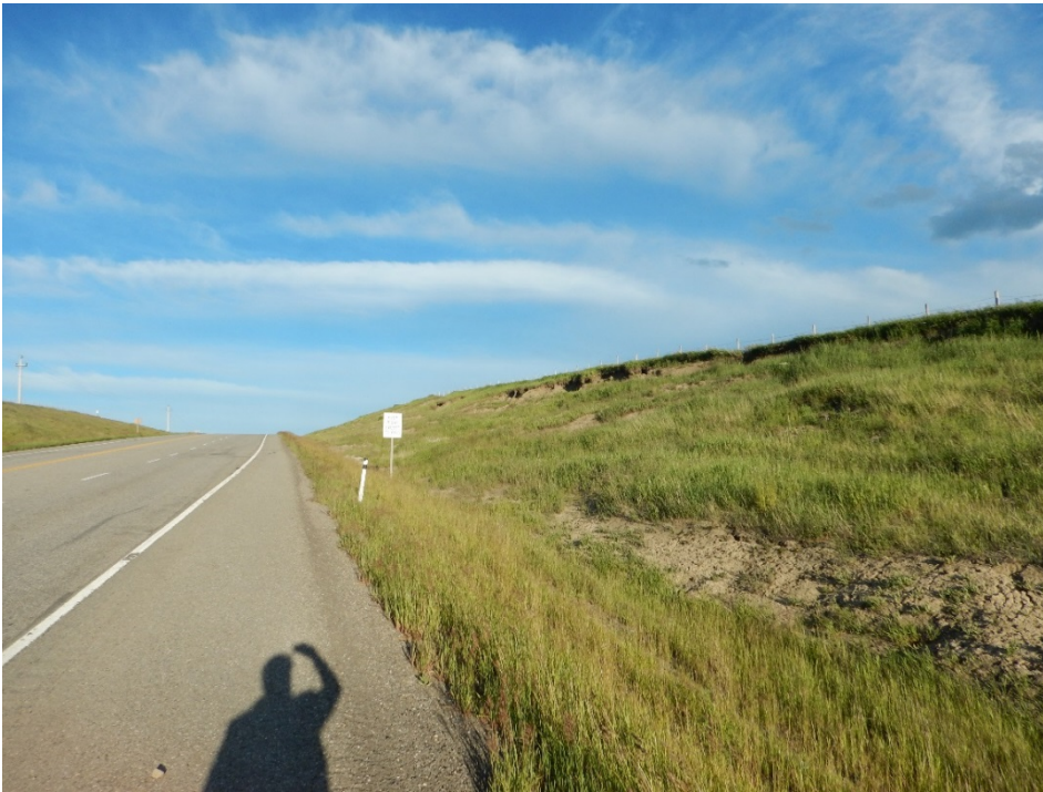
Photo 4 Looking southeast at the failing back slope. The photo was taken on June 15, 2016.
