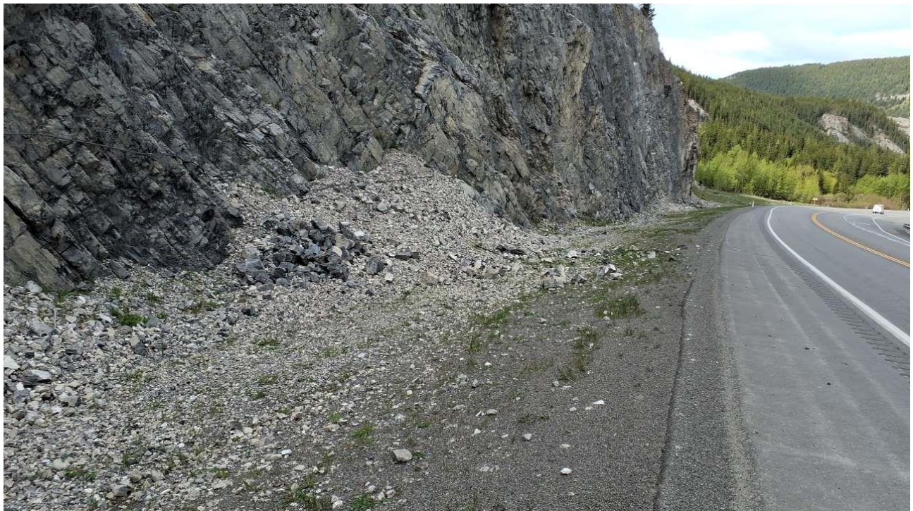
Photo 4 Rock fall debris at the base of the wire mesh and ditch along the rock slope. Photo was taken facing west on May 30, 2024.
