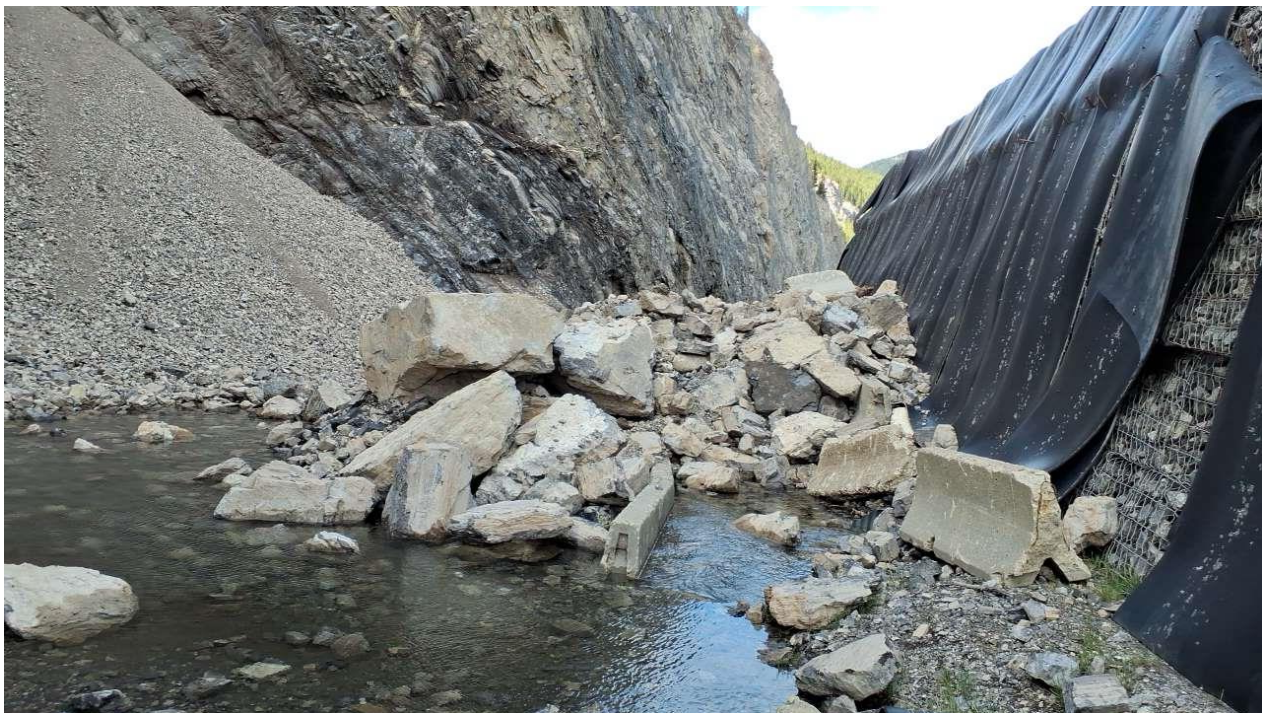
Photo 6 Debris accumulated behind gabion barrier. Photo was taken facing west on May 30, 2024.
