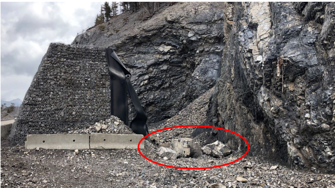
Photo 4 Debris accumulation behind the barrier needs cleaning out (indicated by red circle). Photo was taken on May 20, 2022, facing northeast.
