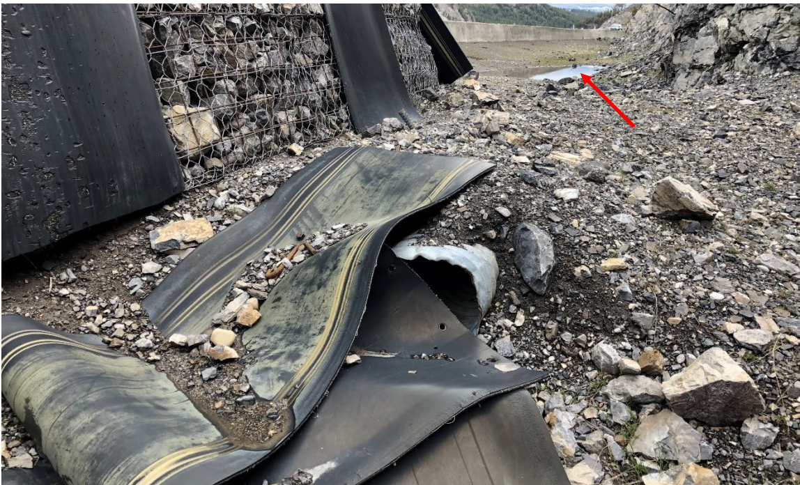
Photo 2 Rockfall material behind the gabion wall is blocking surface water drainage culverts. Standing water near the gabion wall is indicated by red arrow. Photo taken on May 20, 2022, facing northeast.
