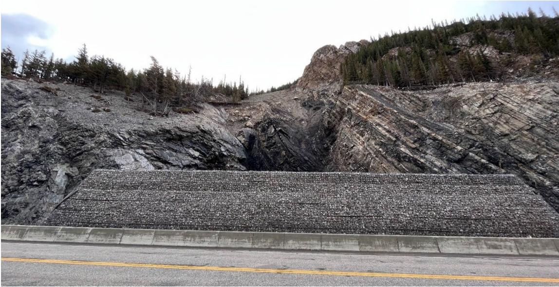
Photo 2 Rockfall material behind the gabion wall is blocking surface water drainage culverts. Standing water near the gabion wall is indicated by red arrow. Photo taken on May 20, 2022, facing northeast.
