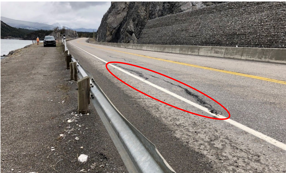
Photo 6 Longitudinal pavement cracking in the north (westbound) lane (indicated by red circle). Photo taken on May 20, 2022, facing northeast.
