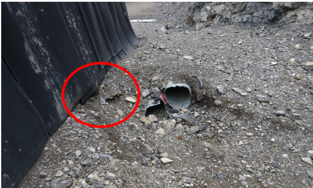
Photo 2 Rubber mats to protect gabion wall from damage. Erosion is occurring at toe of wall (red circle) and could undermine the wall. Photo taken facing east on May 10, 2019.
