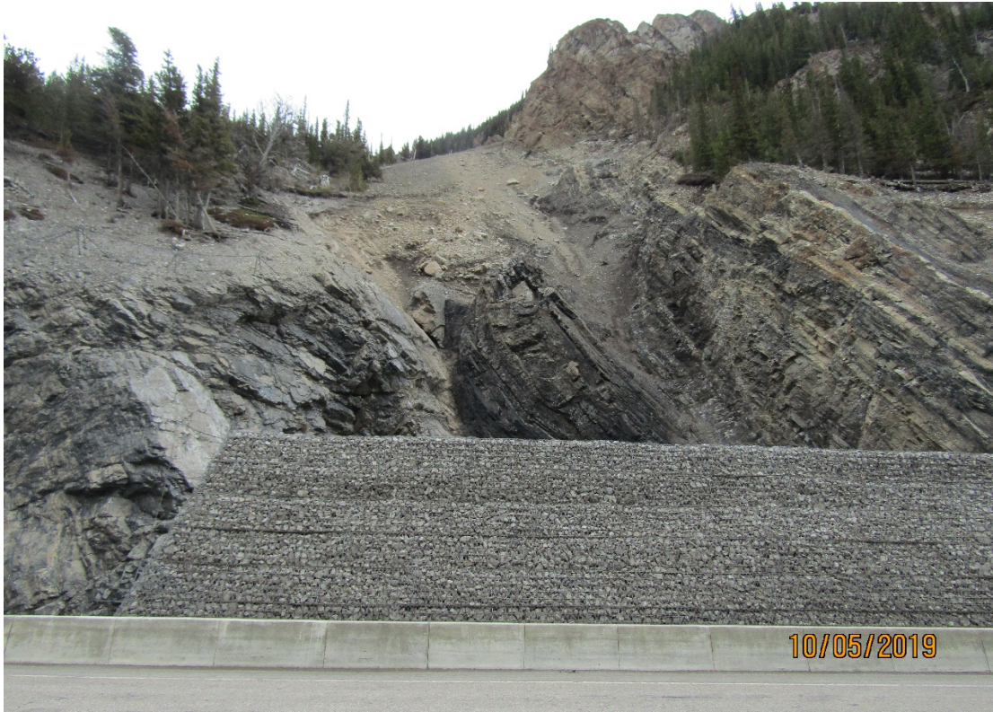
Photo 2 Rubber mats to protect gabion wall from damage. Erosion is occurring at toe of wall (red circle) and could undermine the wall. Photo taken facing east on May 10, 2019.
