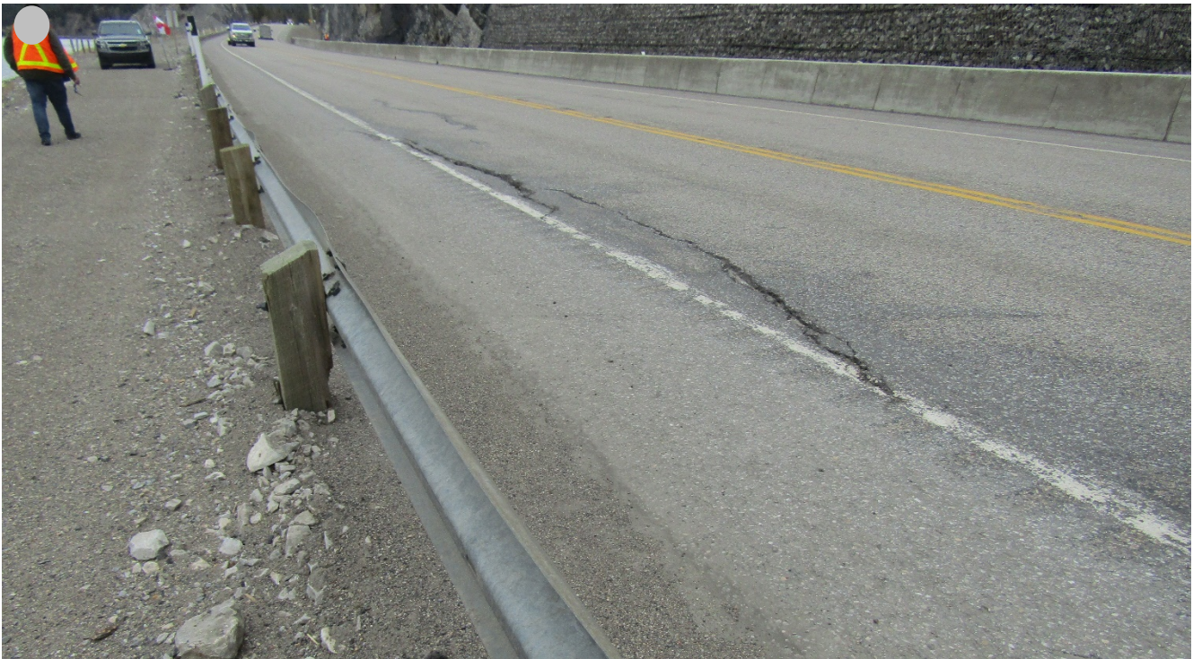
Photo 6 Pavement cracking adjacent to the lake. Photo taken facing east on May 10, 2019.
