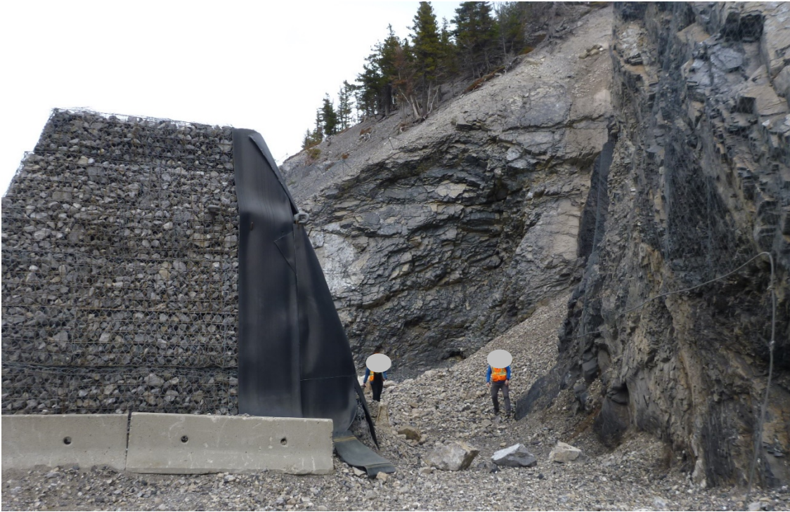
Photo 4 Mesh covered rock slope to the southeast of the barrier. Photo was taken facing east on May 10, 2019.
