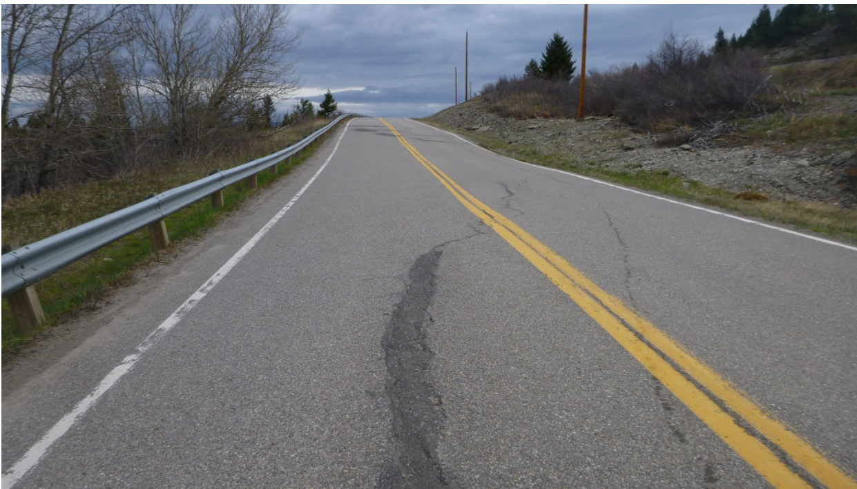
Photo 2 West flank of landslide zone. Note crack sealing on pavement. Photo taken facing southwest on May 10, 2019.
