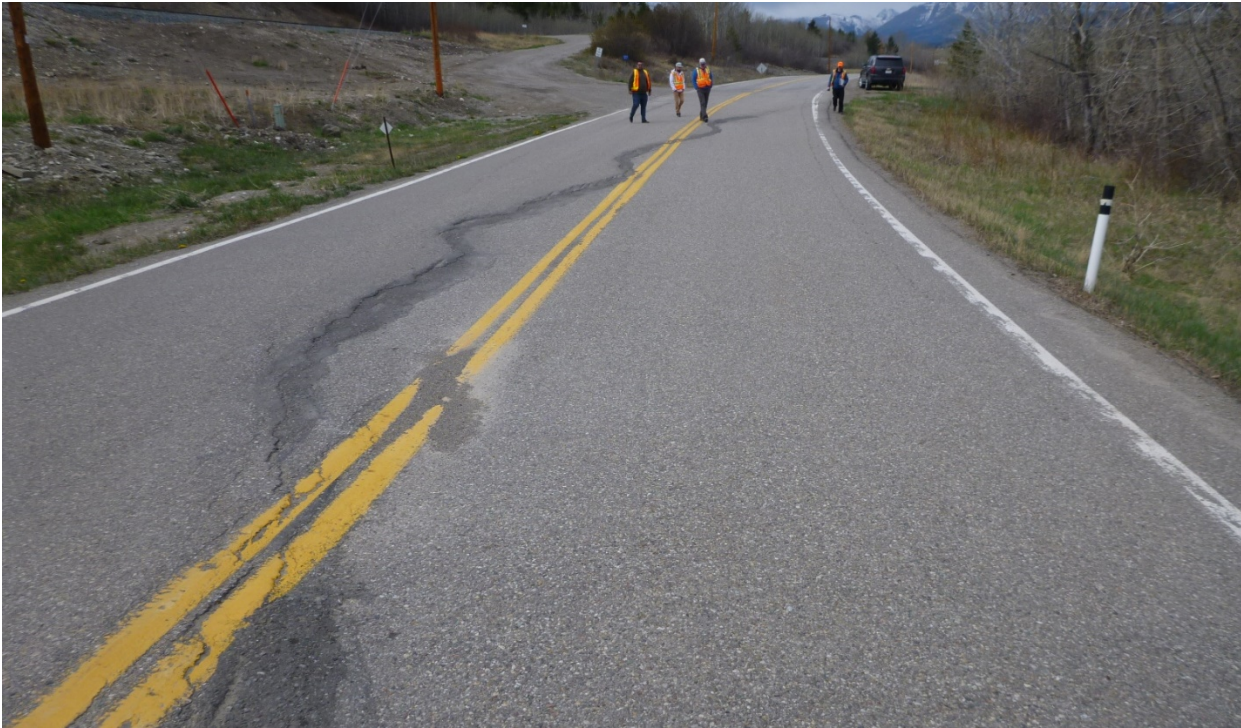
Photo 2 West flank of landslide zone. Note crack sealing on pavement. Photo taken facing southwest on May 10, 2019.
