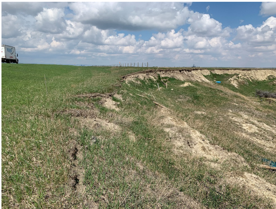
Photo 2 Head scarp located up to 5 m past the fence line. Photo taken facing north on May 10, 2023.
