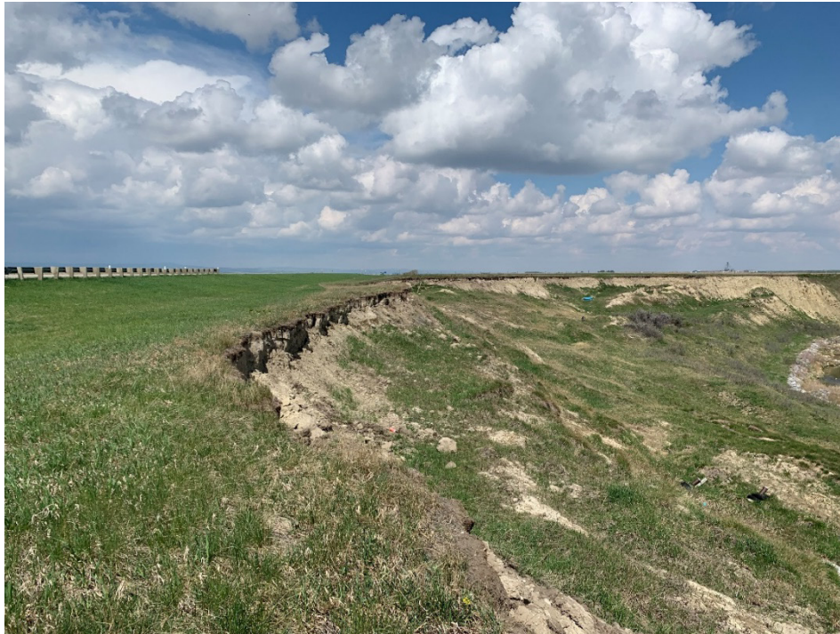
Photo 4 Ongoing slide movement retrogressing towards the highway. Photo taken facing southeast on May 10, 2023.
