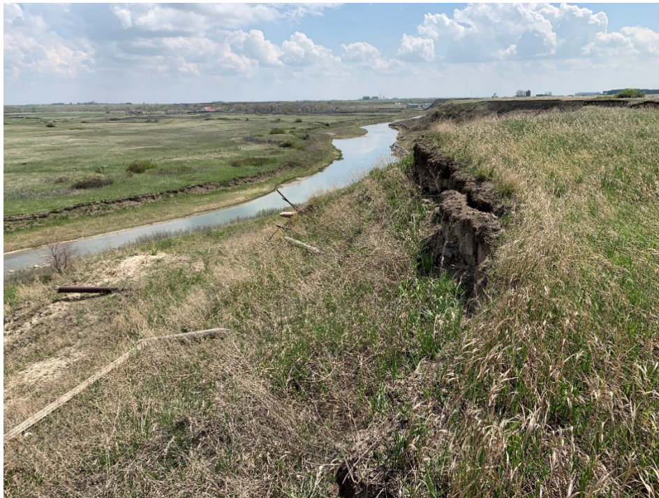
Photo 4 Ongoing slide movement retrogressing towards the highway. Photo taken facing southeast on May 10, 2023.
