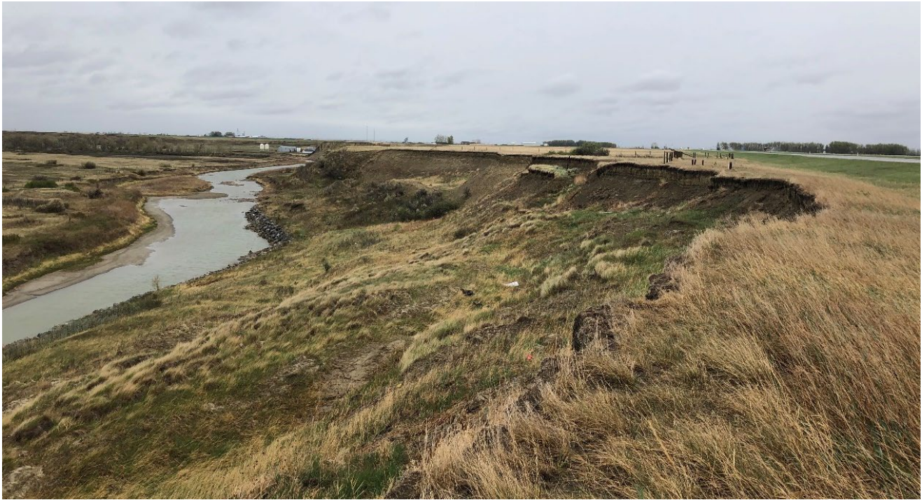
Photo 4 The head of the slide is retrogressing towards the highway. Photo taken May 19, 2022 facing south.
