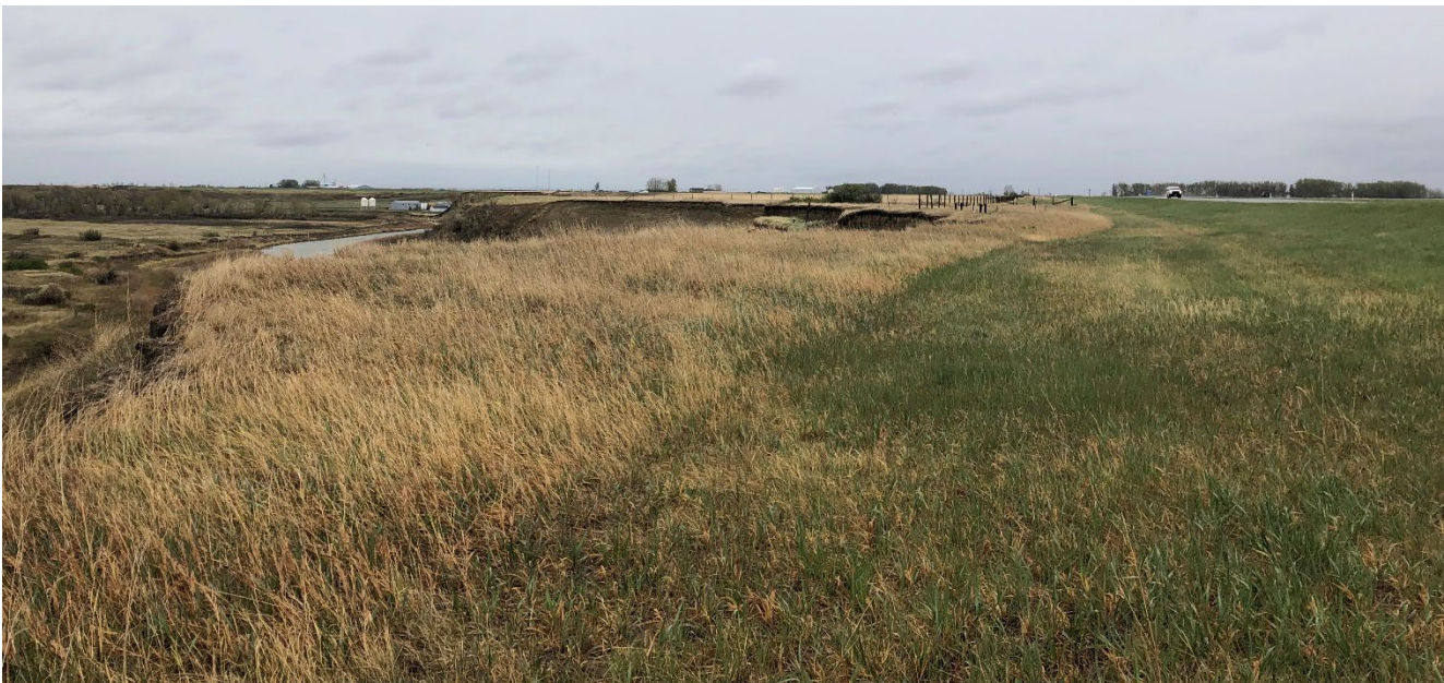
Photo 4 The head of the slide is retrogressing towards the highway. Photo taken May 19, 2022 facing south.
