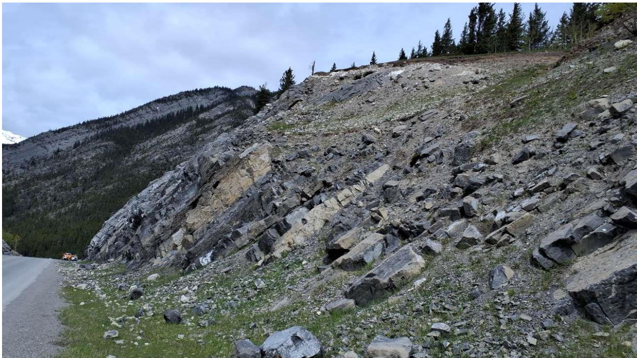
Photo 6 South end of Site B. Loose rock with the potential to fall into the ditch. Photo taken on May 27, 2024 facing northwest.
