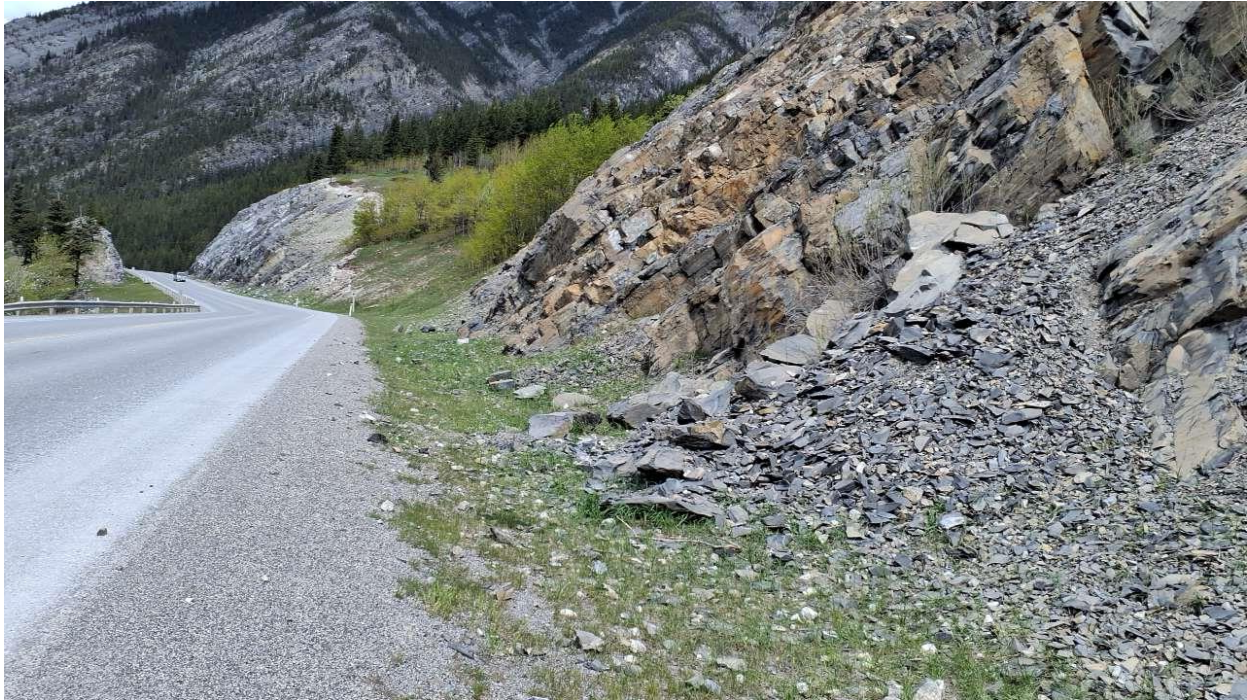
Photo 6 South end of Site B. Loose rock with the potential to fall into the ditch. Photo taken on May 27, 2024 facing northwest.
