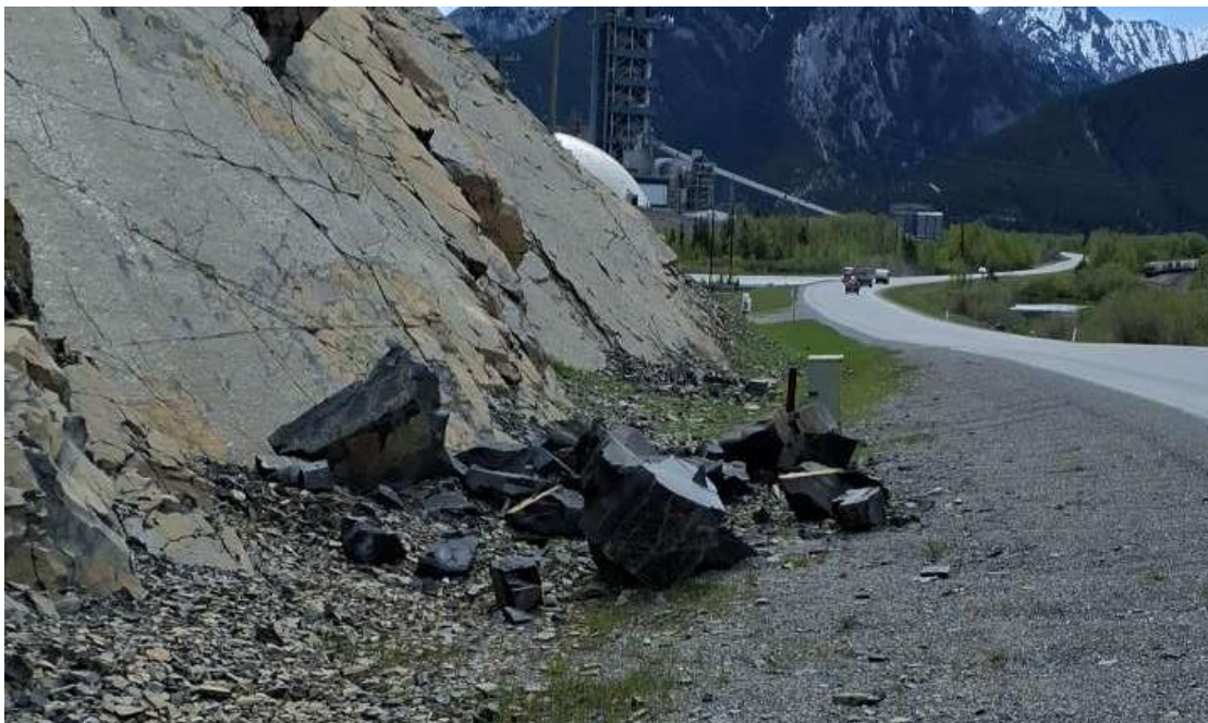
Photo 2 The north (westbound) ditch at Site A, recent rockfall debris in ditch at the south end of the site. Photo taken on May 27, 2024, facing southeast.
