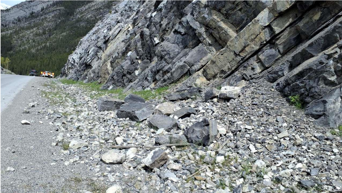
Photo 7 North end of Site B. Rockfall debris in ditch (unchanged from 2022). Photo taken on May 27, 2024 facing northwest.
