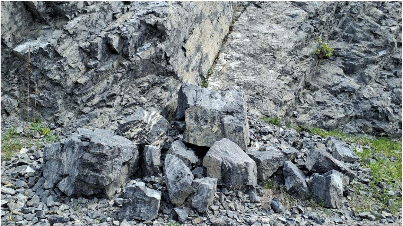
Photo 7 North end of Site B. Rockfall debris in ditch (unchanged from 2022). Photo taken on May 27, 2024 facing northwest.
