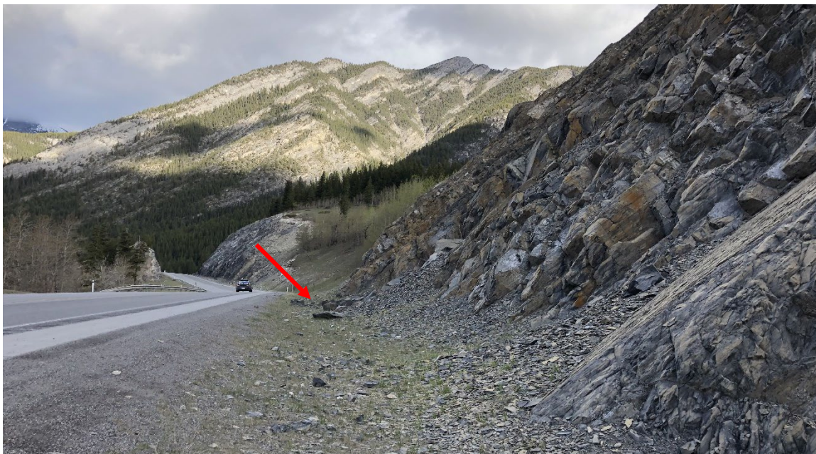
Photo 2 The north (westbound) ditch at Site A is relatively flat and some rockfall debris was observed at the toe of the slope (larger debris indicated by red arrow). Photo taken May 17, 2022, facing southeast.
