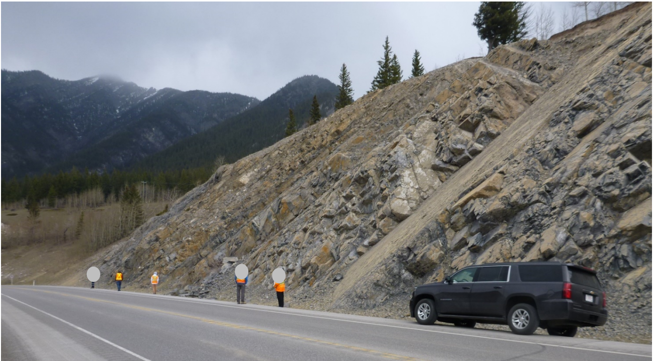
Photo 4 Adversely dipping bedrock at Site B. Photo taken facing north on May 7, 2019.
