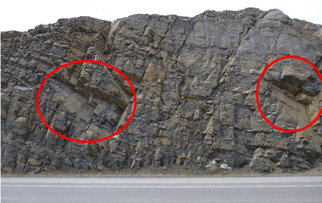
Photo 6 Near vertical rock cut slope at Site A (south of the highway). Areas of historic block failure are shown by red circles. Photo taken facing west on May 7, 2019.
