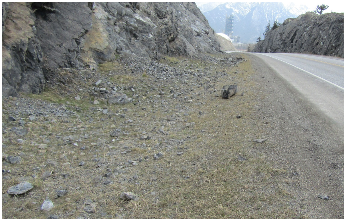
Photo 8 Rockfall in catchment ditch at Site B. Photo taken facing east on May 7, 2019.
