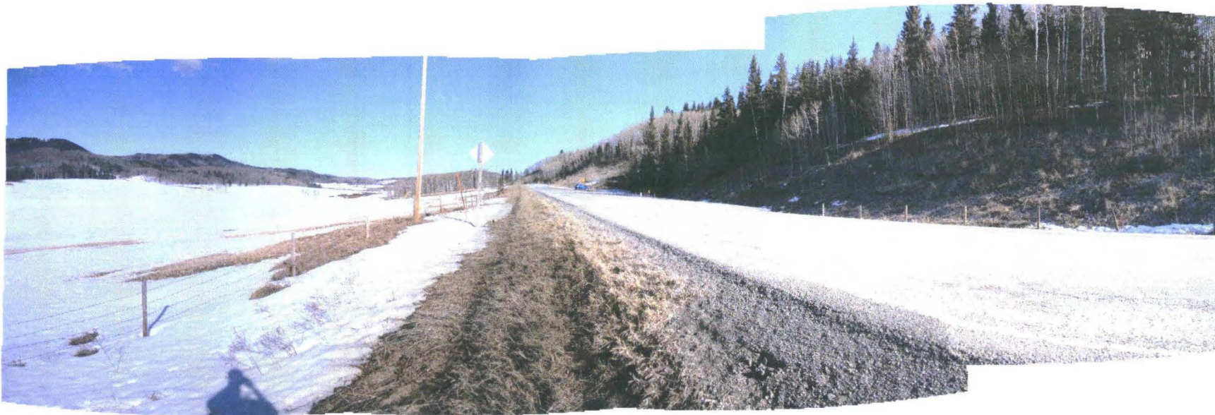
Photograph 2 – Stitched photographs of the site area, facing northbound and taken from the west edge of the road, showing the natural slope downslope of the road, and the cut slope in the ridge upslope of the road.
