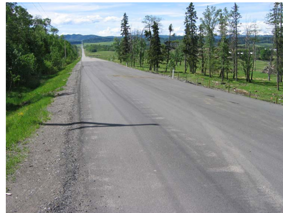
Photo S10(B)-1 (upper left) – May 2006 – facing south along the road. The area was repaved since the 2005 inspection. Minor longitudinal cracking visible in the repaved surface.
