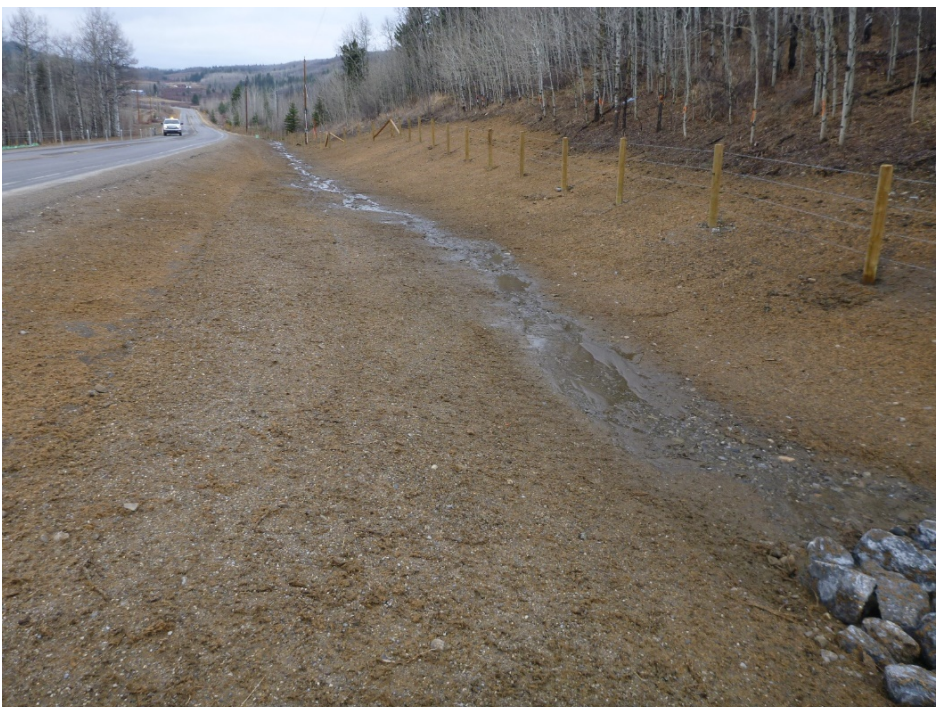
Photo 4 East side of highway ditch. Some erosion noted. Rolled erosion control product not used on ditch bottom. Vegetation not established on slopes. Photo taken facing northeast on April 30, 2018.
