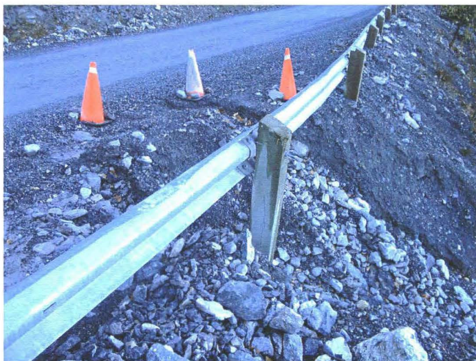
Photo 742-34 (bottom) – Another view of the head of the gully erosion, showing how the guardrail posts have been undermined.
