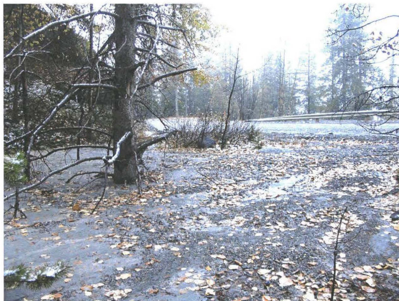
Photo 742-15 (bottom) – Another view of the infilled drainage draw at ~Km 4.1.
