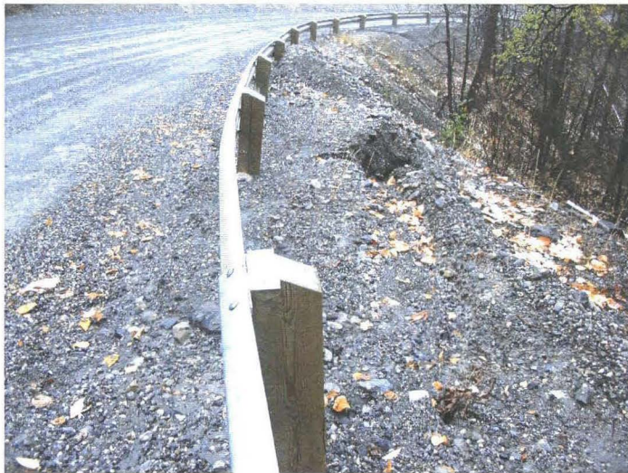
Photo 742-11 (top) – At approximately Km 4.2, showing the ditch flow spilling across the road. Please refer to Photo 742-12 for a view of the head of the erosion gully being formed where this surface runoff flows below the guardrail and onto the fill slope below the road.
