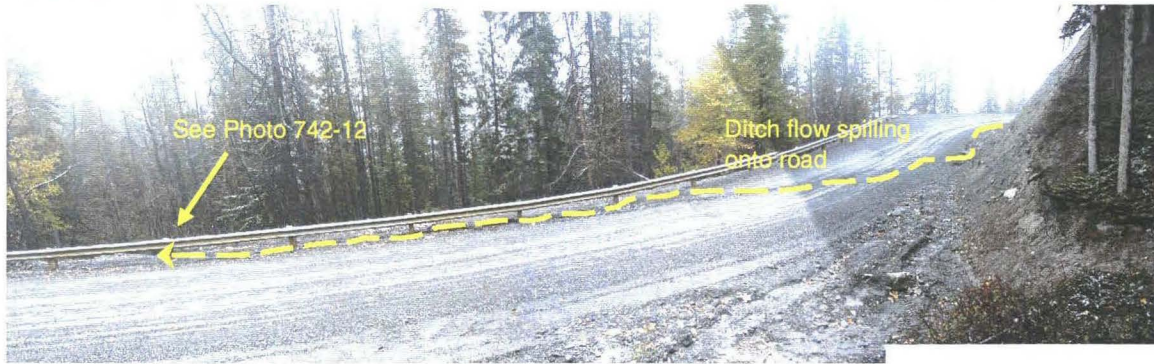
Photo 742-11 (top) – At approximately Km 4.2, showing the ditch flow spilling across the road. Please refer to Photo 742-12 for a view of the head of the erosion gully being formed where this surface runoff flows below the guardrail and onto the fill slope below the road.
