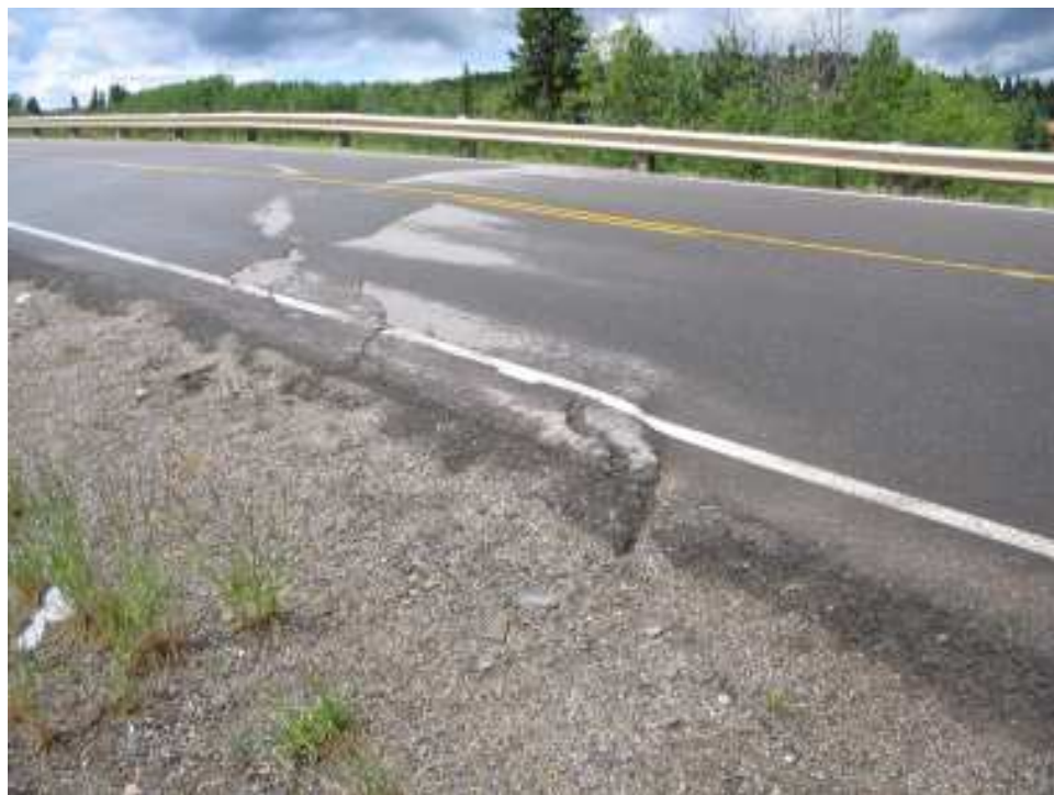
Photo S7-3 – June 2007 (lower left) Facing northwest across the diagonal crack and downdrop area around Sta. 5+280/5+290. At the time of the inspection, the road surface to the east of the crack (right hand side of photo) was downdropped approximately 30 to 50 mm relative to the west side.
