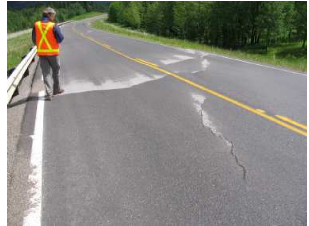
Photo S7-1 – June 2007 (upper left) Facing east across the area where a pronounced diagonal crack and downdrop of the road surface was observed around Sta. 5+280/5+290 in the 2007 inspection. This area is approximately 120 m west of where the shear keys were installed in 2004 to mitigate landslide damage to the road surface. The crack position is marked with the orange “Sharp Shoulders” sign on the south side of the road and the vertical displacement across the crack is visible in the guardrail profile.
