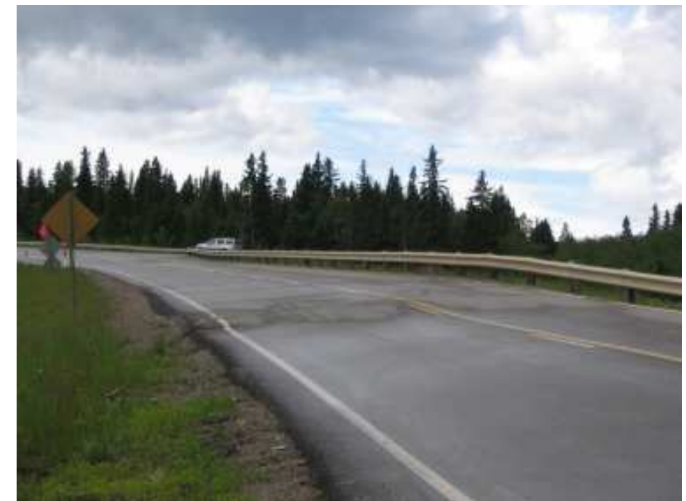
Photo S7-3 – June 2007 (lower left) Facing northwest across the diagonal crack and downdrop area around Sta. 5+280/5+290. At the time of the inspection, the road surface to the east of the crack (right hand side of photo) was downdropped approximately 30 to 50 mm relative to the west side.
