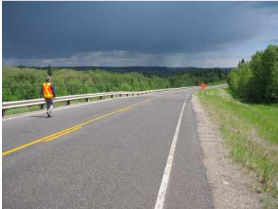
Photo S7-1 – June 2007 (upper left) Facing east across the area where a pronounced diagonal crack and downdrop of the road surface was observed around Sta. 5+280/5+290 in the 2007 inspection. This area is approximately 120 m west of where the shear keys were installed in 2004 to mitigate landslide damage to the road surface. The crack position is marked with the orange “Sharp Shoulders” sign on the south side of the road and the vertical displacement across the crack is visible in the guardrail profile.
