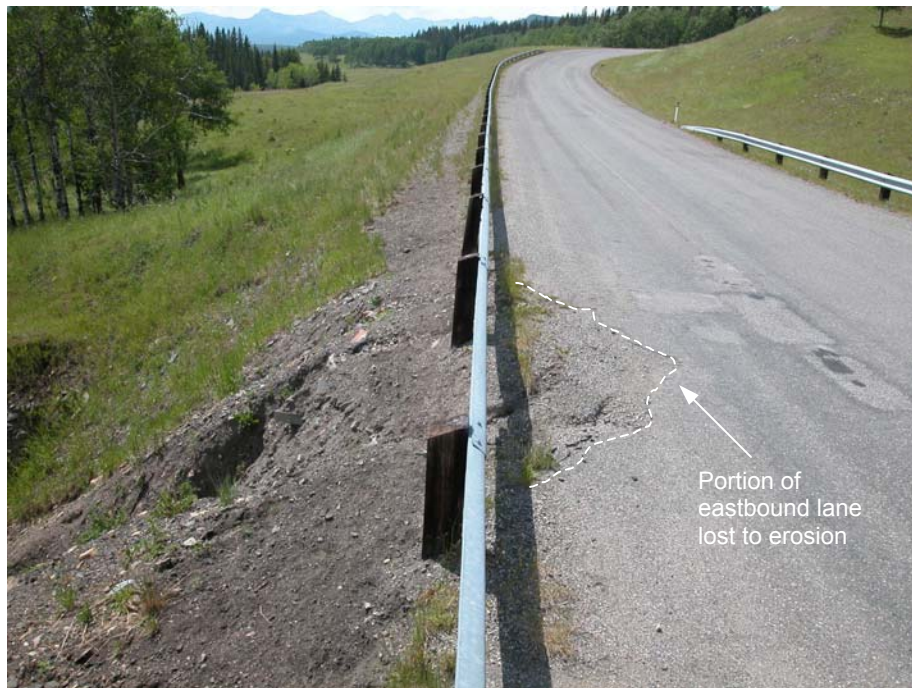
Photo 2 (lower left) Facing west along the south guardrail. The gully erosion in the fill slope below the guardrail is visible, along with some erosion and settlement of the pavement surface along the south edge of the road.
