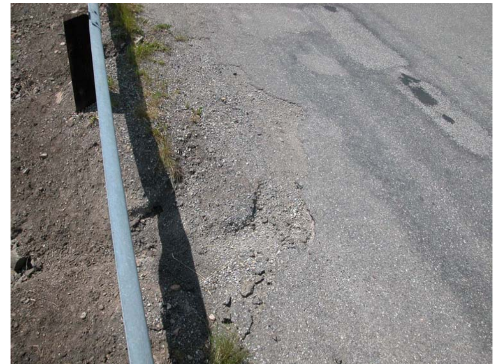
Photo 2 (lower left) Facing west along the south guardrail. The gully erosion in the fill slope below the guardrail is visible, along with some erosion and settlement of the pavement surface along the south edge of the road.
