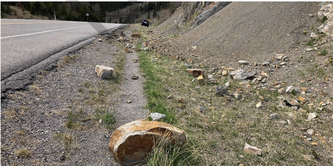
Photo 2 Rockfall material in the ditch and debris fan on the lower portion of the back slope. Photo taken May 16, 2022, facing west.
