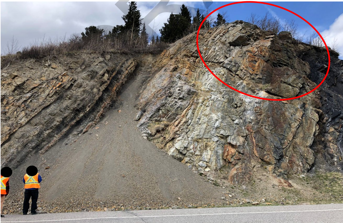
Photo 4 Large debris fan in central portion of the slope. Block adjacent to debris fan (indicated by red circle) is at risk of detaching. Photo taken May 16, 2022, facing north.
