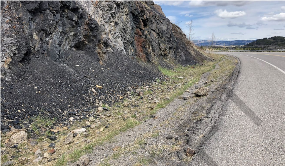
Photo 4 Large debris fan in central portion of the slope. Block adjacent to debris fan (indicated by red circle) is at risk of detaching. Photo taken May 16, 2022, facing north.
