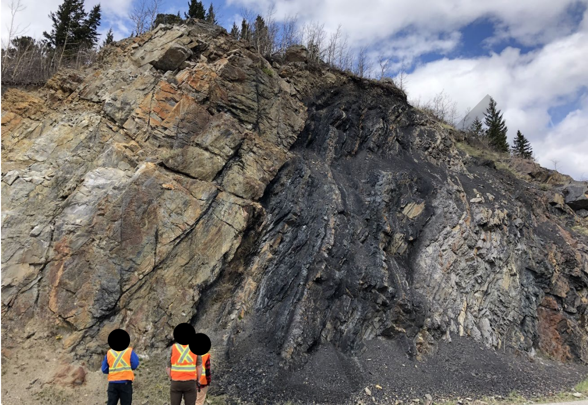
Photo 2 Rockfall material in the ditch and debris fan on the lower portion of the back slope. Photo taken May 16, 2022, facing west.
