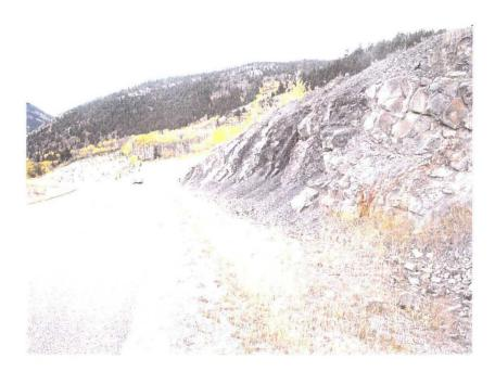
Photo 2 (bottom) – Facing west across the West of Fir Creek Rock Cut site. The accumulated rockfall debris along the toe of the slope should be cleaned in order to restore the full capacity of the ditch and maintain the low Consequence Factor for this site.
