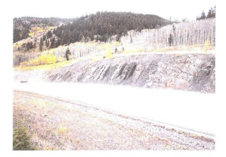
Photo 1 (top) – Facing north across Highway 541 towards the West of Fir Creek Rock Cut site. The exposed rock at this site is generating ongoing minor rockfalls of gravel to cobble sized debris. The existing ditch appears to be sufficient to prevent debris from landing on the road.
