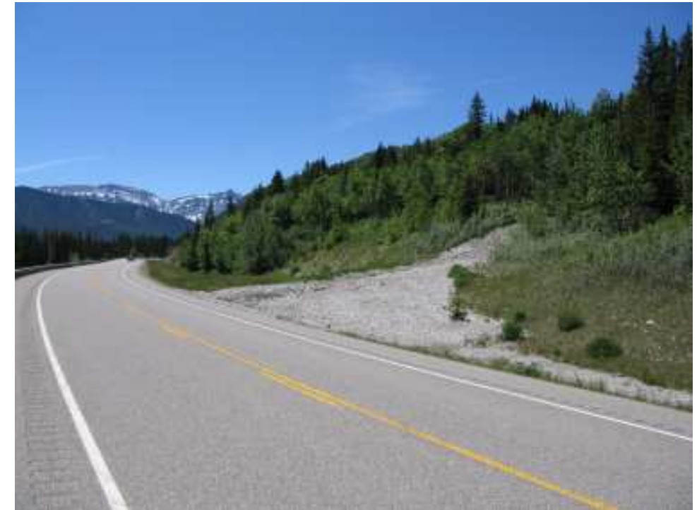
Photo S21-2 – June 2007 (upper left) Facing westbound along the highway with the 2004 debris flow deposit visible on the upslope side of the road.
