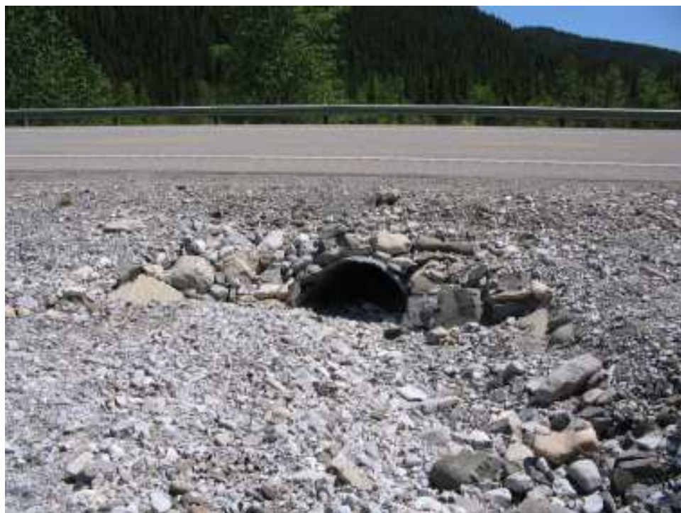
Photo S21-3 – June 2007 (upper right) Facing downstream towards the inlet of the 1250 mm diameter culvert below the highway. The culvert inlet is in roughly the same condition as noted in the August 2005 inspection and is approximately 2/3 full of debris.
