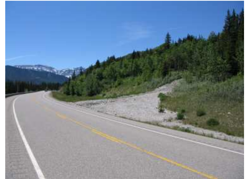
Photo S21-2 – June 2007 (upper left) Facing westbound along the highway with the 2004 debris flow deposit visible on the upslope side of the road.
