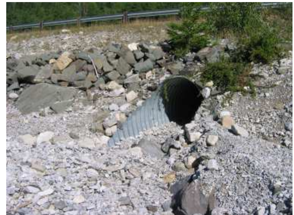
Photo S21-3 – June 2007 (upper right) Facing downstream towards the inlet of the 1250 mm diameter culvert below the highway. The culvert inlet is in roughly the same condition as noted in the August 2005 inspection and is approximately 2/3 full of debris.
