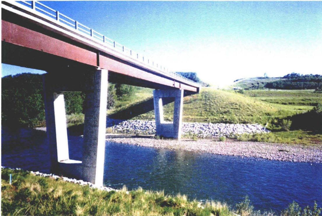
Photo 1 – Looking North at north abutment.
