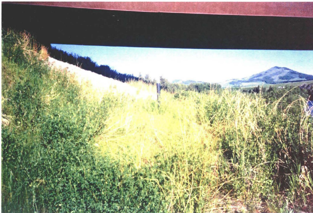
Photo 2 – Looking west at south abutment fill slope.
