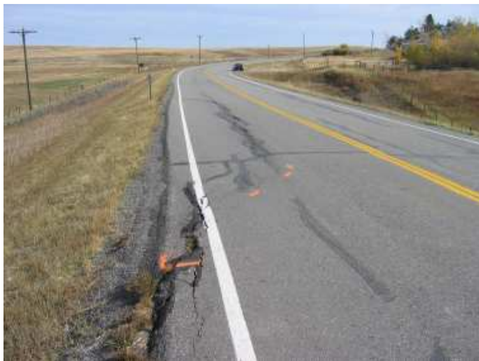
Photo S24-7 – Westbound Lane Site –September 2006 (lower left) Facing northeast across the settlement and cracking area in the westbound lane, as it appeared in September 2006. The semi-circular pattern of the cracking is consistent with a rotational slump failure in the northwest embankment slope (left side of photo), however a corresponding toe bulge below the road was not observed. The linear cracks in the eastbound lane (right hand side of photo) are judged to be unrelated to the circular cracking pattern in the westbound lane.
