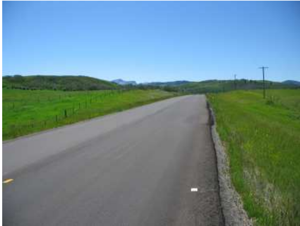
Photo S24-5 – Westbound Lane Site –September 2006 (upper left) Facing southwest across the recently repaved settlement and cracking area in the westbound lane. Compare with Photo S24-6 which shows the damage to this area as it appeared in September 2006 before the recent paving.
