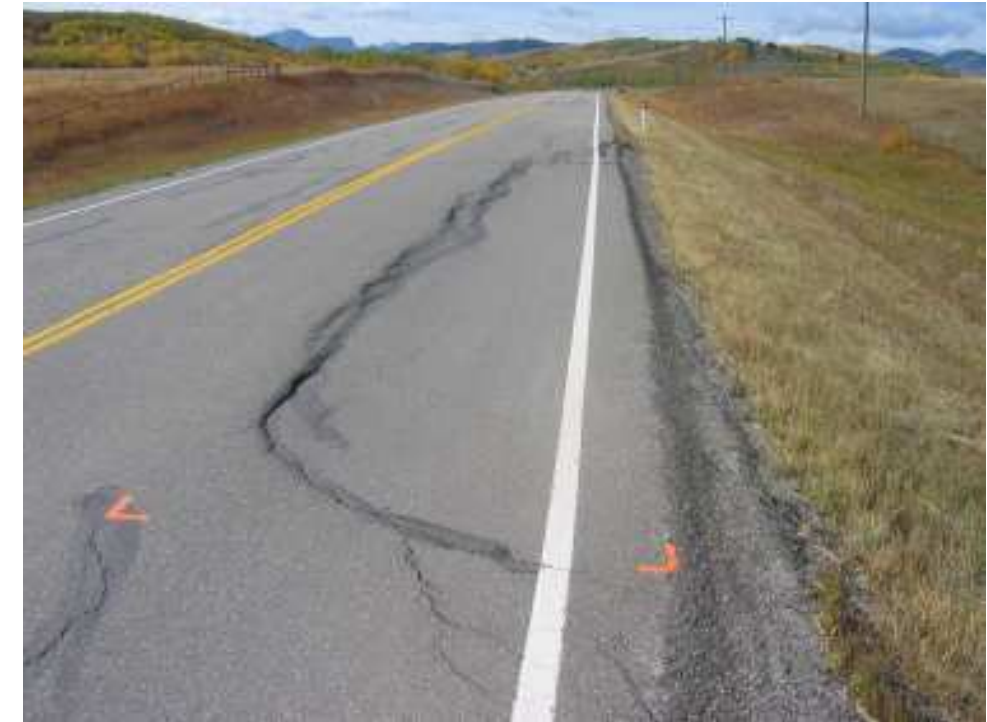
Photo S24-5 – Westbound Lane Site –September 2006 (upper left) Facing southwest across the recently repaved settlement and cracking area in the westbound lane. Compare with Photo S24-6 which shows the damage to this area as it appeared in September 2006 before the recent paving.
