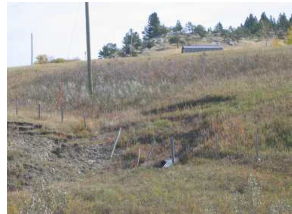
Photo S24-7 – Westbound Lane Site –September 2006 (lower left) Facing northeast across the settlement and cracking area in the westbound lane, as it appeared in September 2006. The semi-circular pattern of the cracking is consistent with a rotational slump failure in the northwest embankment slope (left side of photo), however a corresponding toe bulge below the road was not observed. The linear cracks in the eastbound lane (right hand side of photo) are judged to be unrelated to the circular cracking pattern in the westbound lane.
