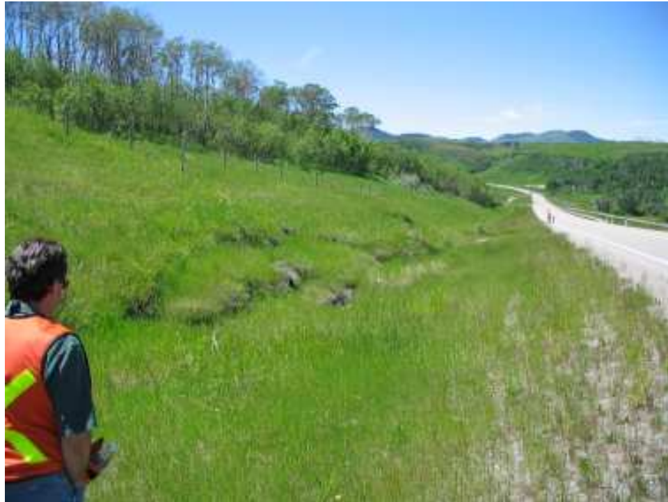
Photo S23-4 – June 2007 (left) Closer view, facing west, across one of the visible toe bulges in the landslide.
