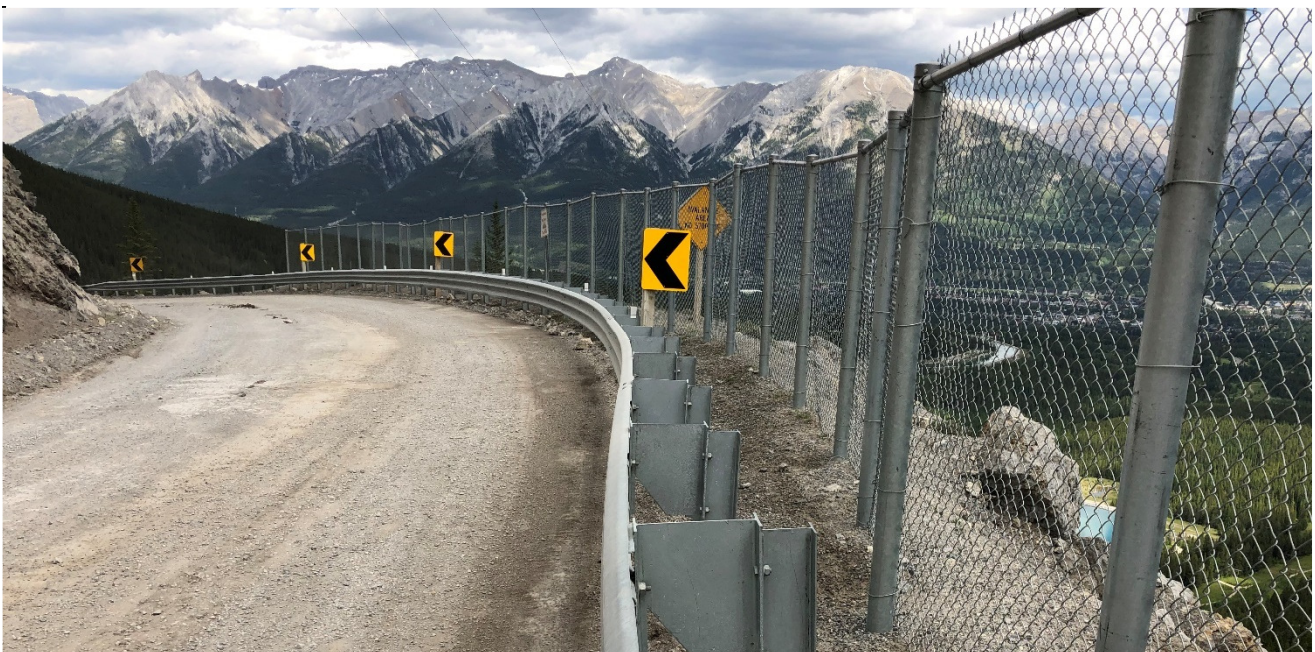
Photo 2 New guard rail barrier and chain link fence after completion of the gabion repairs. Photo taken facing northeast on July 6, 2020.
