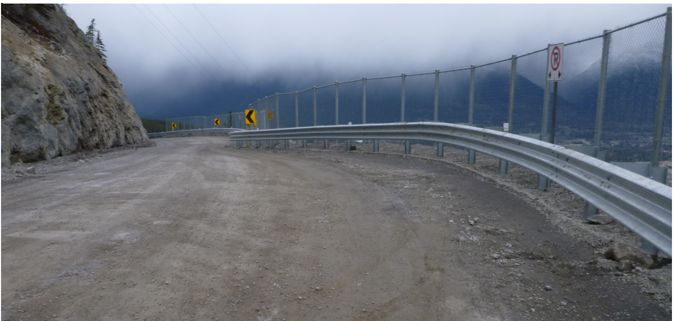
Photo 2 New guard rail barrier and chain link fence after completion of the gabion repairs. Photo taken facing northeast on May 7, 2019.
