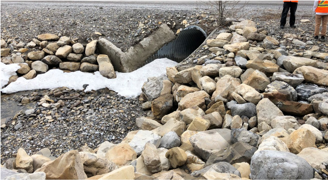
Photo 2 Riprap armoring on the channel upstream of the CSP culvert inlet, on the east side of the highway. Photo taken May 17, 2022, facing southeast.
