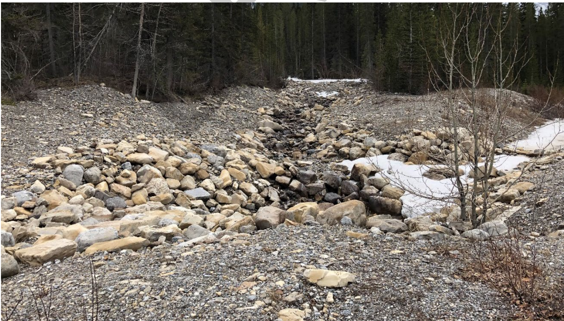
Photo 2 Riprap armoring on the channel upstream of the CSP culvert inlet, on the east side of the highway. Photo taken May 17, 2022, facing southeast.
