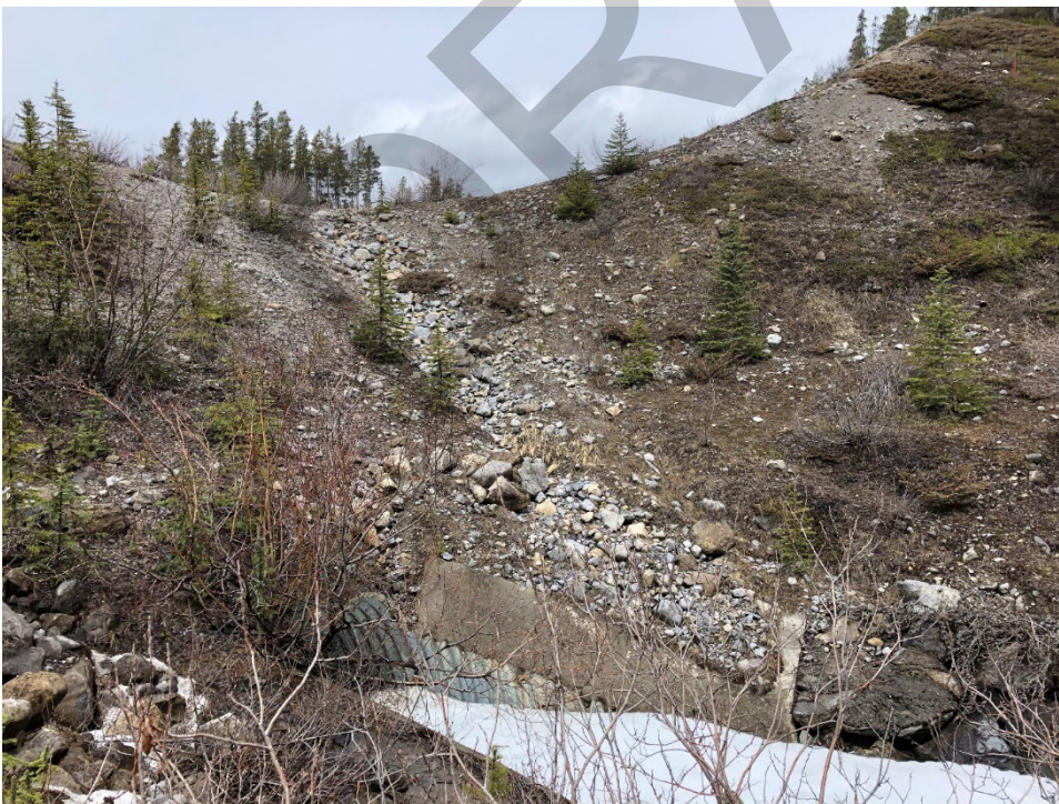
Photo 5 Inlet of the 2 m diameter CSP culvert and east highway embankment slope. Photo taken May 17, 2022, facing north.
