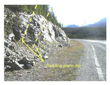
Photo 742-50 (middle) – Facing southbound along the east road ditch and roughly along the strike direction of the bedding in the exposed rock. Note the favorable bedding plane dip relative to the cut slope, i.e. the bedding dips away from the cut slope face. Note also the minor amounts of rockfall debris in the ditch.
