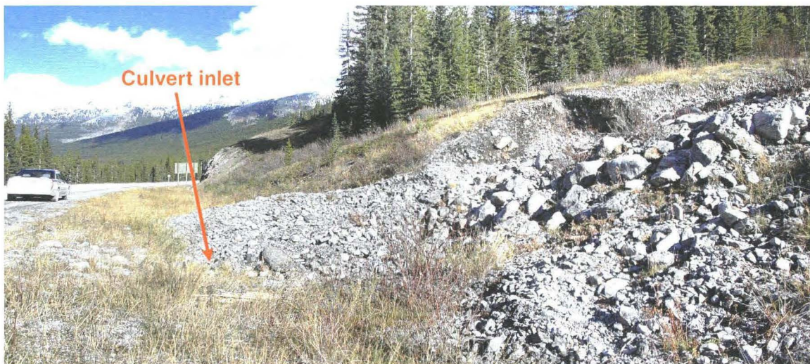
Photo 742-47 (bottom) – Facing northbound along the upslope road ditch. Note the up to boulder-sized material deposited in the upslope road ditch, northbound of the culvert inlet.
