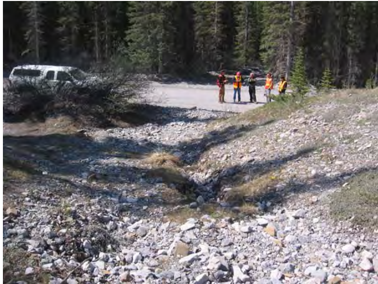
Photo 1 – June 2009 (top) Facing downstream along the creek channel towards the highway crossing. Note the lack of surface flow in the channel.
