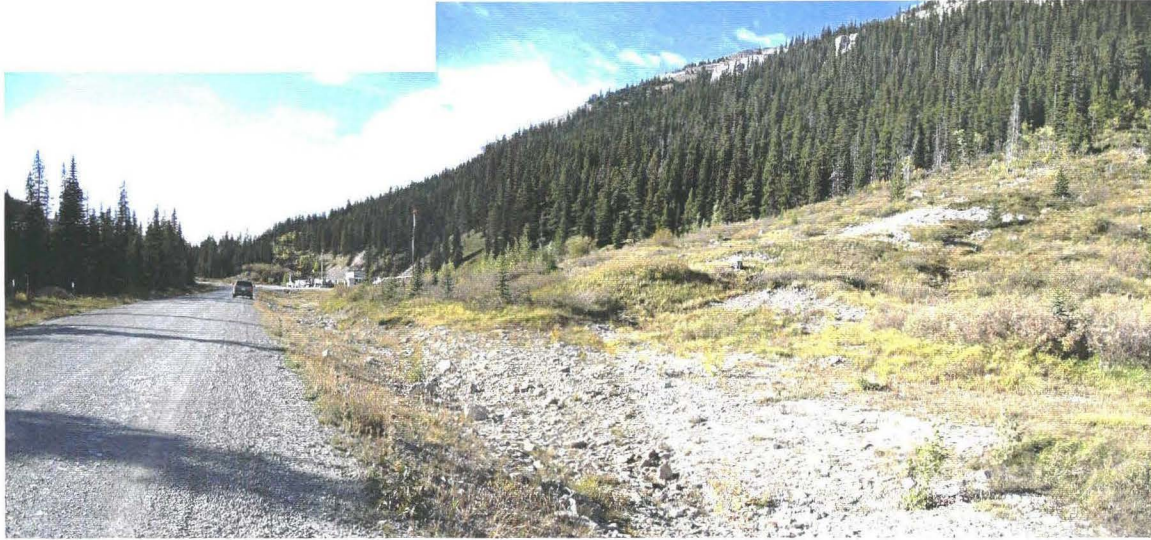
Photo 940-37 (top) – Facing west/northbound across the lower portion of the fan which slopes at 10°. It appears that the lowermost portion of the fan was graded flat for the construction of the highway. There was no active surface creek channel visible on the fan at the time of the site inspection.
