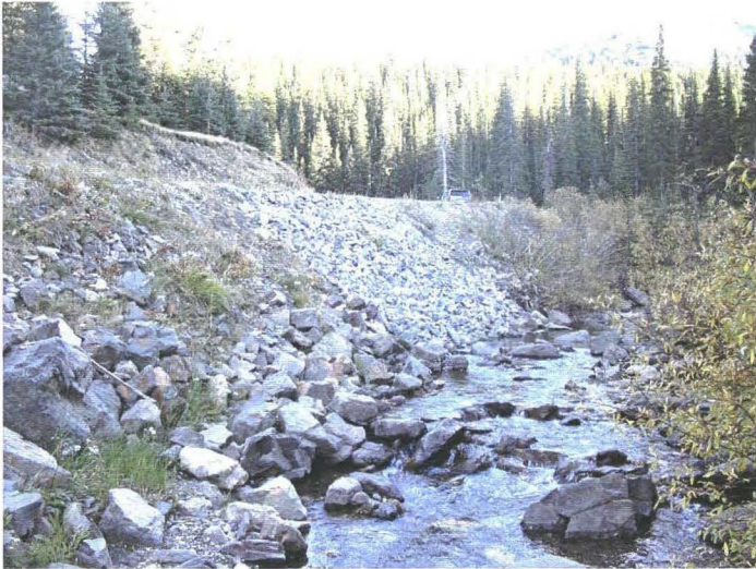
Photo 940-47 (bottom) – Facing upstream along the creek, towards the 2008 repair area.
