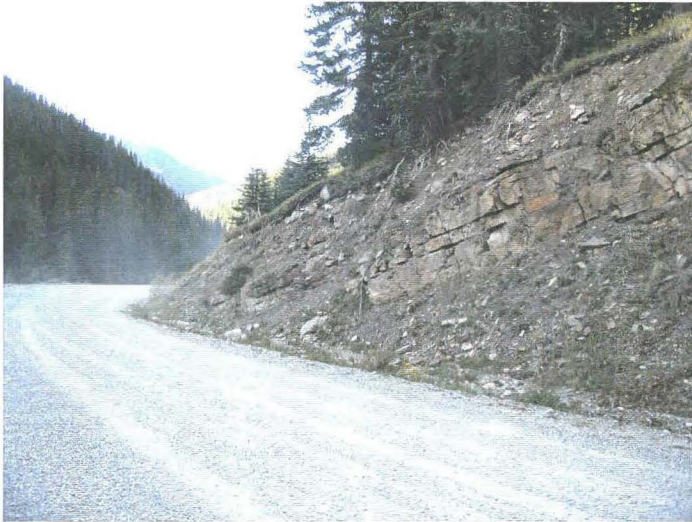
Photo 940-42 (top) – General view of the cut slope, facing northbound.
