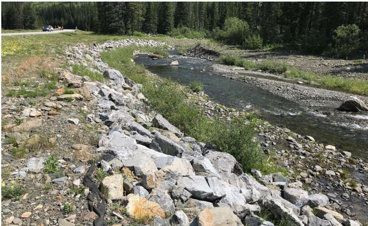
Photo I-14 S068-5: Repaired and riprap lined bank of Wilkinson Creek after 2013 washout. Photo was taken facing northwest on July 9, 2021.
