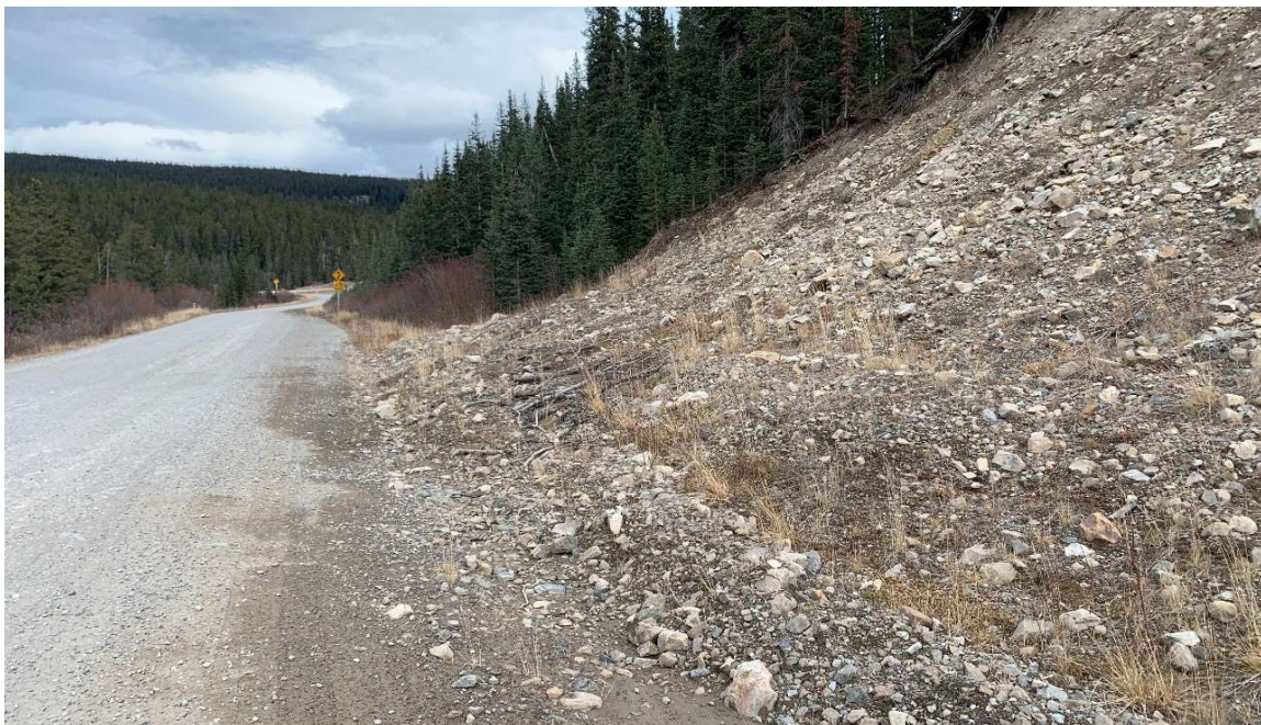
Photo I-2 S068-1: Accumulation of gravel at the back slope toe due to surface erosion and weathering. Photo was taken facing east on October 22, 2021.
