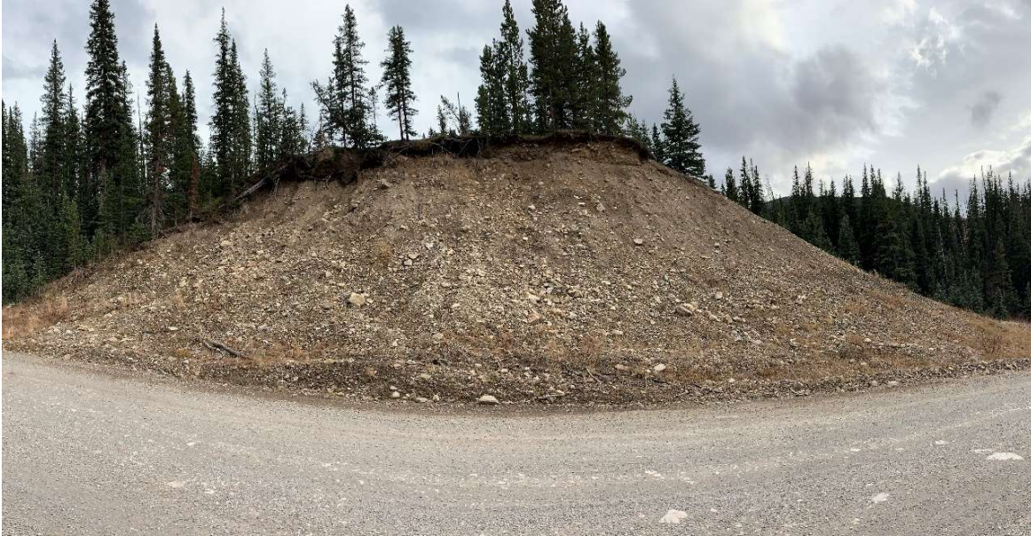
Photo I-2 S068-1: Accumulation of gravel at the back slope toe due to surface erosion and weathering. Photo was taken facing east on October 22, 2021.
