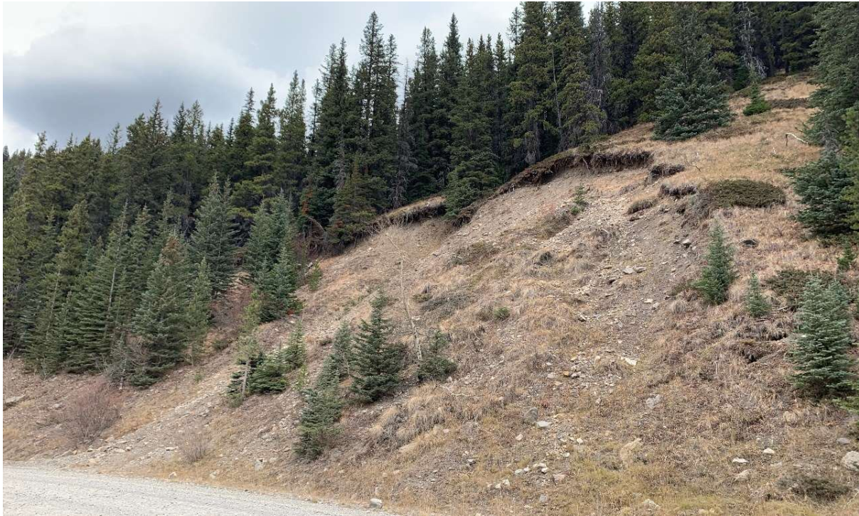
Photo I-10 S068-4: Surface runoff leading to a debris cone at toe of back slope that reduces the available ditch capacity. Photo taken facing north on October 22, 2021.
