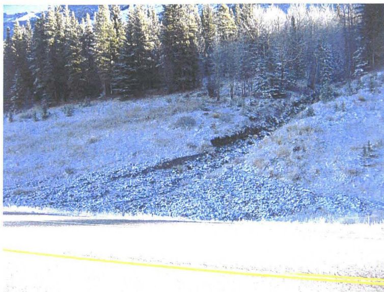
Photo 1 (top) – Fan of debris that has been deposited along the upslope (east) side of Highway 40 at an unnamed creek crossing approximately 500 m north of the Fortress Junction service station. The debris consisted of cobble to boulder sized rocks that appeared to have washed down along the creek channel during peak flows earlier in 2005.
