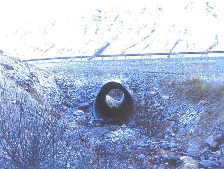
Photo 2 (middle) – Facing downstream through the culvert at the Ripple Rock Creek crossing. Note the lack of debris along the portion of the channel immediately upstream of the culvert inlet.
