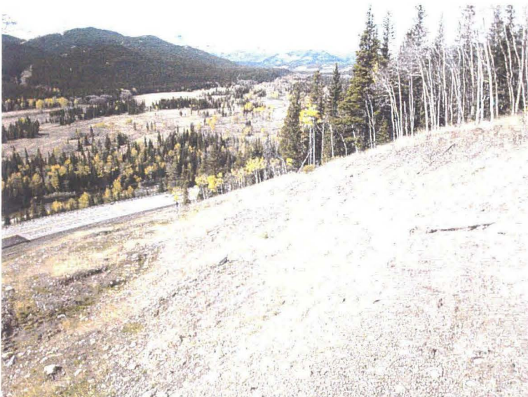
Photo 3 (bottom) – Facing west across the area shown in Photo 2, illustrating the relative position of the slump scarps in the upper portion of the cut slope and the highway.
