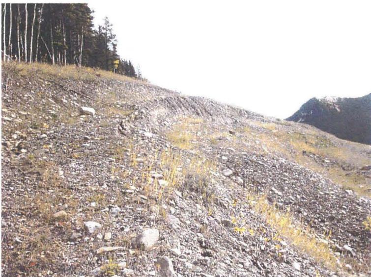
Photo 2 (middle) – Facing east along one of the visible slump scarps near the crest of the cut slope above the road. The slump scarp and vertical dropdown of the slump block is well-defined in the slope profile, however the overall visual appearance does not indicate recent significant movement of the slump block.
