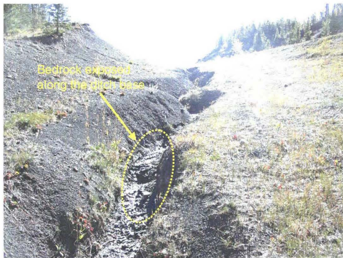
Photo 940-20 (middle) – Facing upstream along the eroded segment of the east road ditch. Further downcutting along this segment of the ditch appears to be limited by the bedrock exposed along the base of the ditch.
